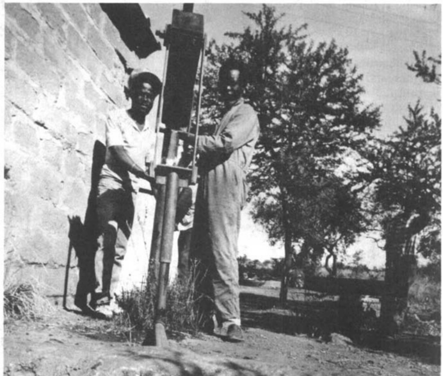
Contract workers will often exclude the community from headwork construction.
