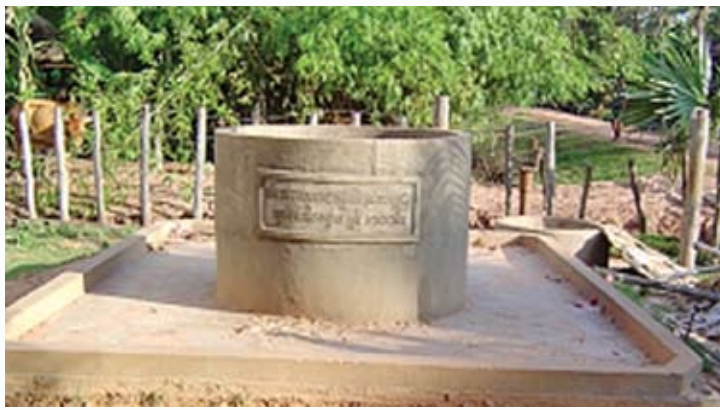
Figure 2.2: Two dug wells with platform and headwall CIPS: Unprotected CSES: Protected
