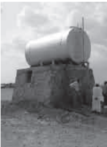
Mogoraib Water Tank
