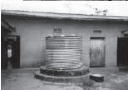
A galvanised steel tank
