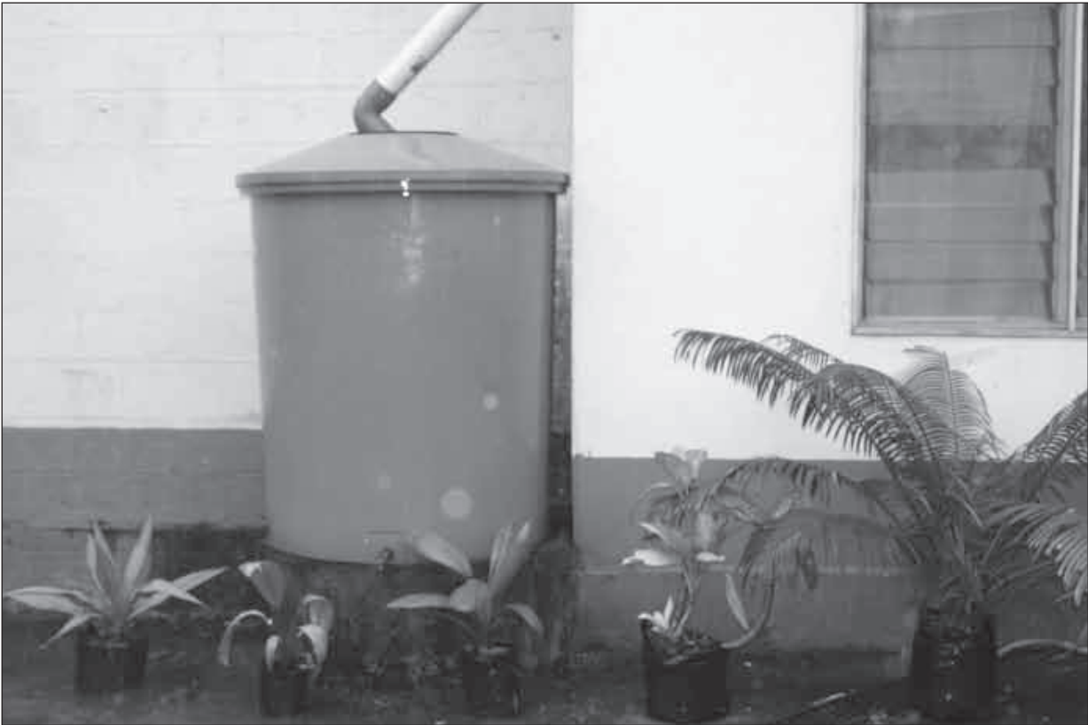
Figure 6: Collecting rainfall in a rain water tank
