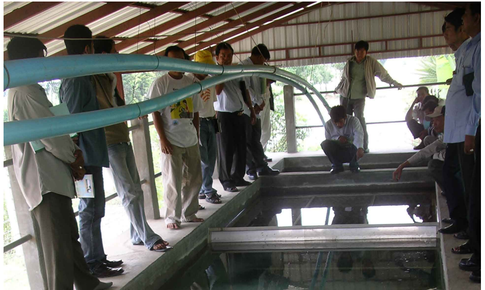
A water treatment plant in rural Cambodia
