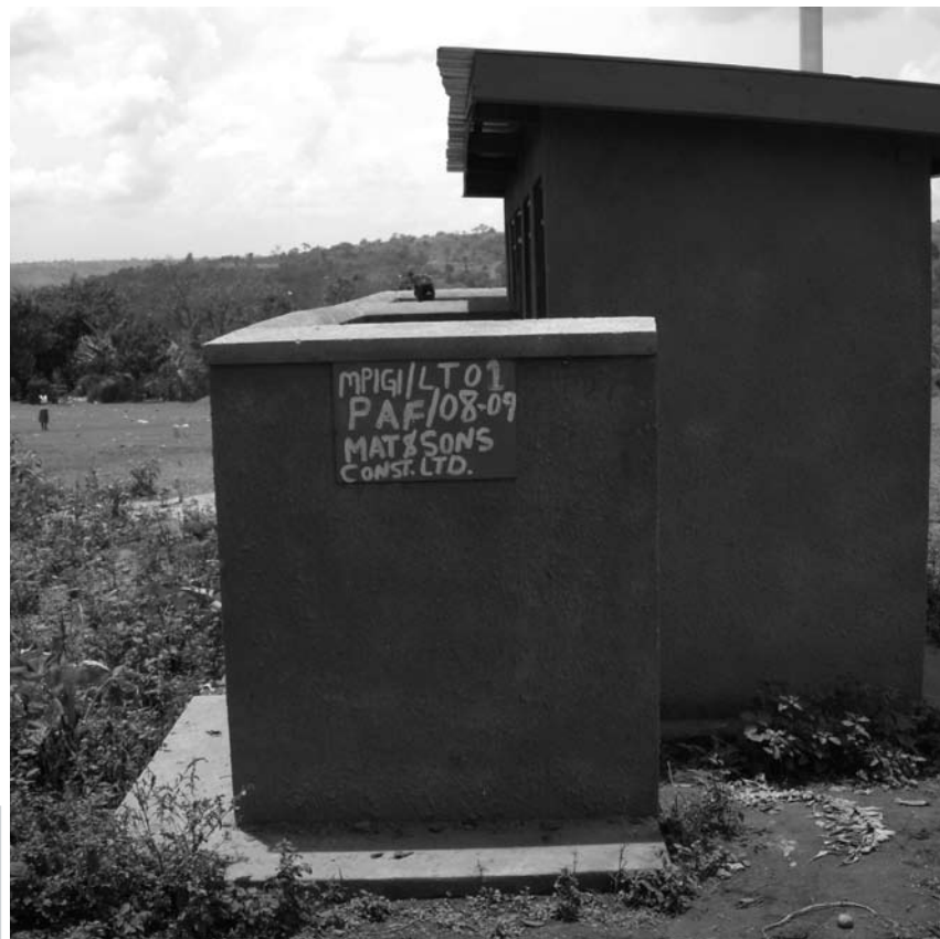
Up-grading of sanitation, using district grants, Mpigi District, September 2009,
