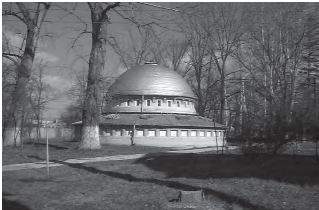
Plate 48. The superstructure of the first well used for water supply in Timișoara, Romania, completed in 1914 (Photo: Aquatim – Water and Sewerage Company of Timișoara).
