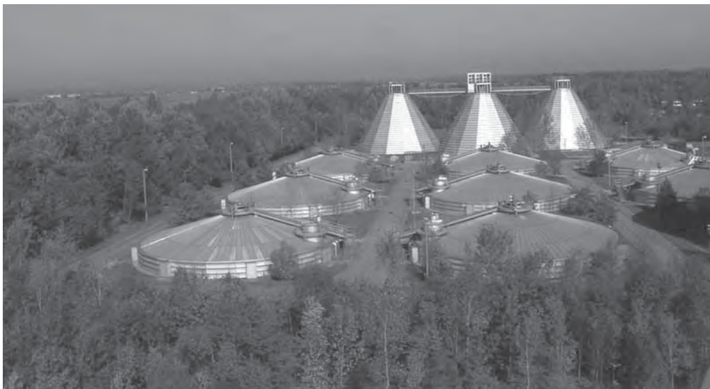
Plate 17. Aerial view of the sludge treatment at the wastewater treatment plant of “Gut Marienhof” constructed from 1986 to 1989 in Munich, Germany — foreground six covered sludge thickeners, in the background three anaerobic digesters, and on the right edge gas storage tank. The plant has one million people equivalent treatment capacity (Photo: Munich Municipal Wastewater Works, 2003)
