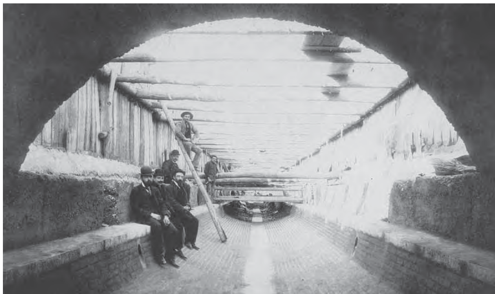
Plate 29. Construction of sewage collector (“collettore”) in the Nosedo area, Milan, Italy, in early 1900s (Photo: Gentile & al. 2003, p. 112; with the permission of Commune of Milan)
