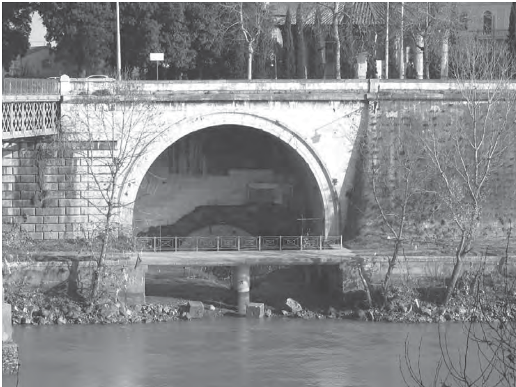
Plate 31. Cloaca Maxima, the first main sewer of Rome built originally for land drainage around 600 BC (Photo: T. Katko, 2005)
