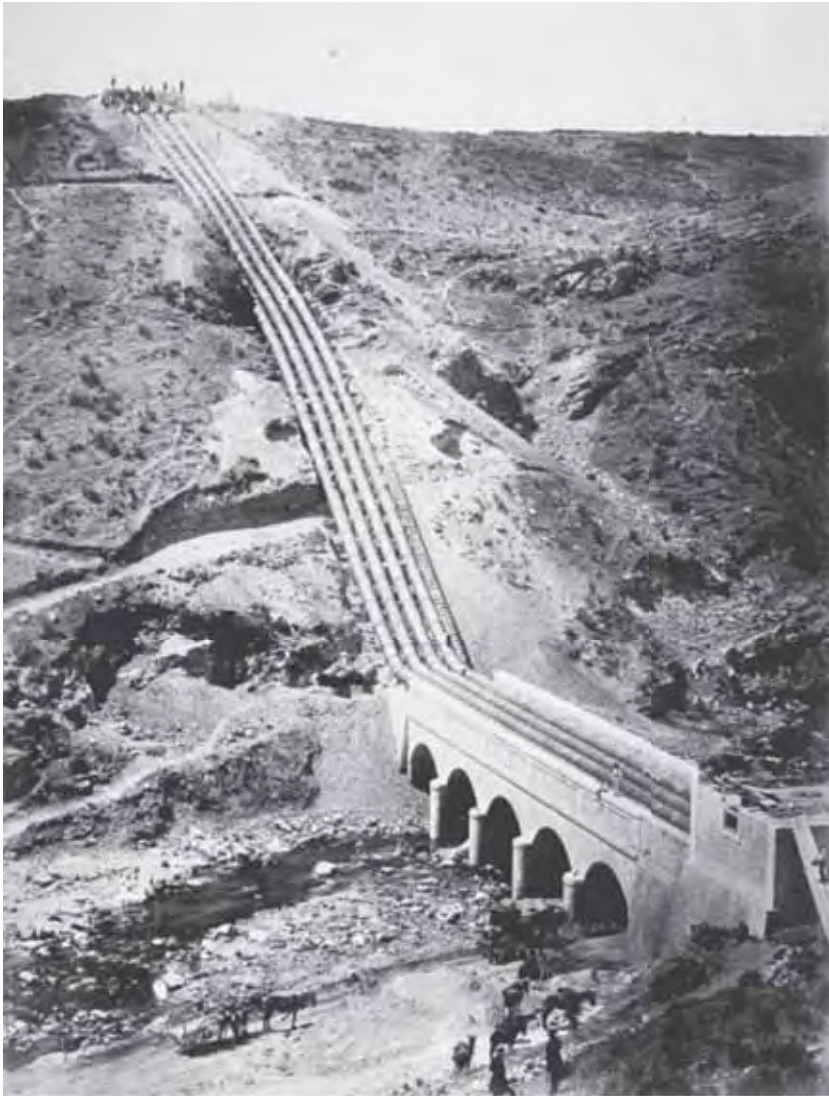
Plate 52. The historic Sifon de Guadalix constructed for water supply in Madrid in 1858 (Photo: Canal de Isabel II)
