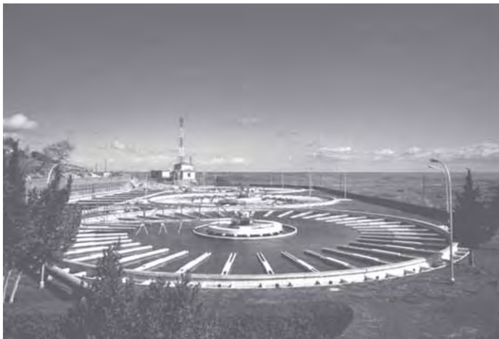
Plate 53. ETAP de Torrelaguna, water treatment plant of Madrid, Spain, completed in 1967 (Photo: M. Angel Gómez, Canal de Isabel II).
