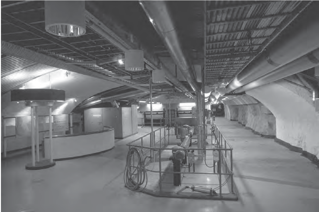
Plate 59. Entrance of the Henriksdal wastewater treatment plant located underground in Stockholm, Sweden. The plant has 700,000 people equivalent treatment capacity (Photo: Thomas Henrikson, Orange AV-Produktion)
