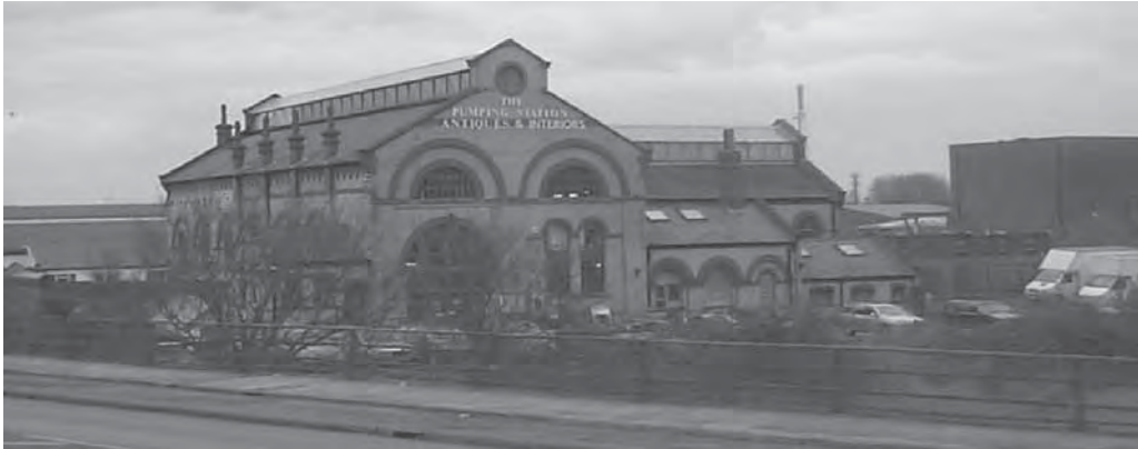
Plate 62. Sewage pumping station circa 1880 in Cardiff, Wales, pumping sewage to a tank sewer discharging to the sea on the outgoing tide. Nowadays used as an Antique & Craft Centre (Photo: Dwr Cymru Welsh Water)
