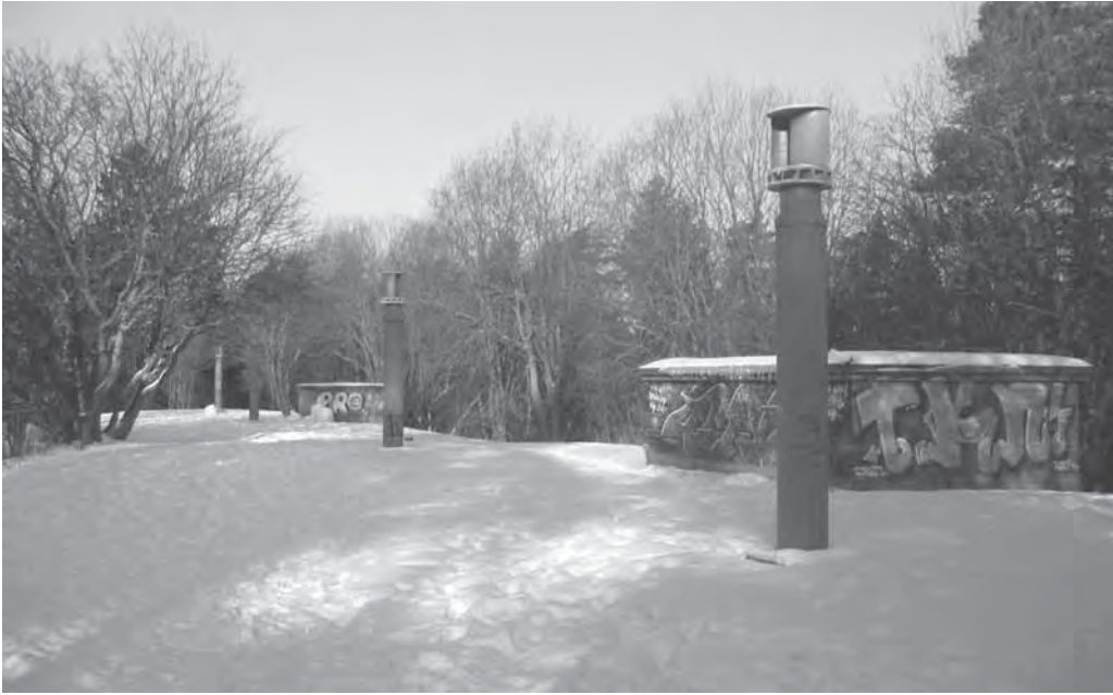
Plate 10. Underground high-level water reservoir in the Pyynikki eskar in Tampere, Finland — constructed in 1898, still in use in 2005 (Photo: P. Juuti, 2005)
