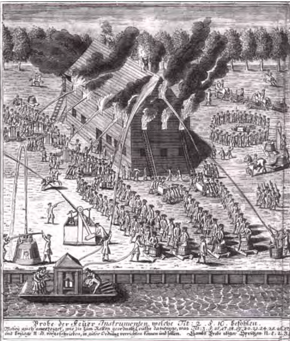
Plate 14. Fire-fighting in Berlin, Germany, illustration from 1727 (Photo: Bärthel 1997, p. 27; with the permission of Berlin Wasser)
