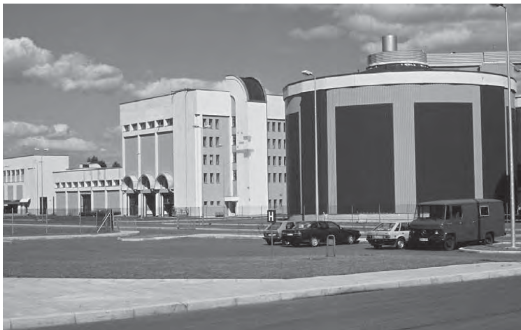
Plate 35. Wastewater treatment plant of Kaunas, Lithuania, taken into use in 1999 (Photo: P. Pietilä 2002)
