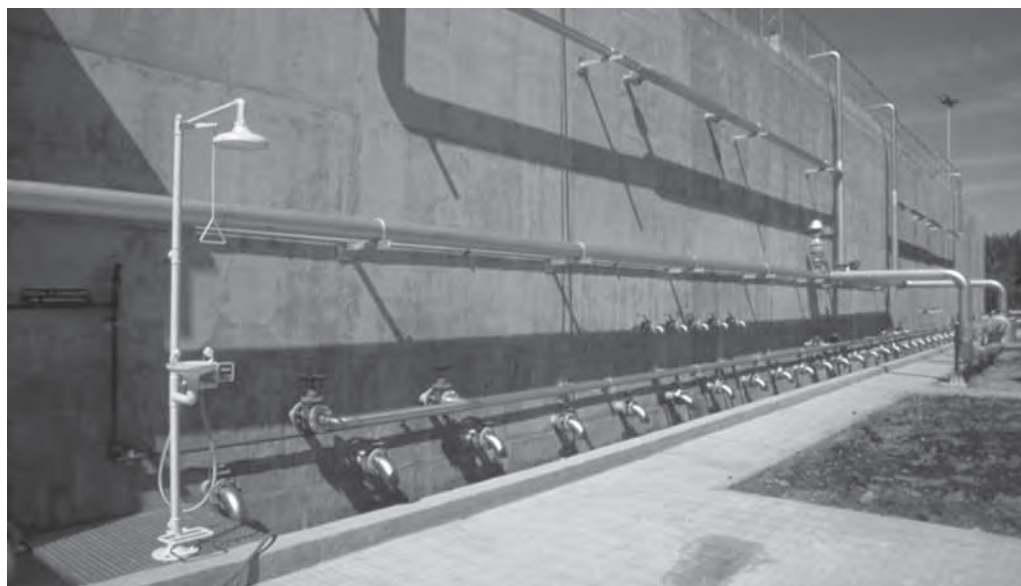
Plate 50. Plant based on anaerobic UASB process in Córdoba, Spain for combined treatment of municipal and yeast factory wastewaters. Purge and net of gas in front (Photo: EMACSA)
