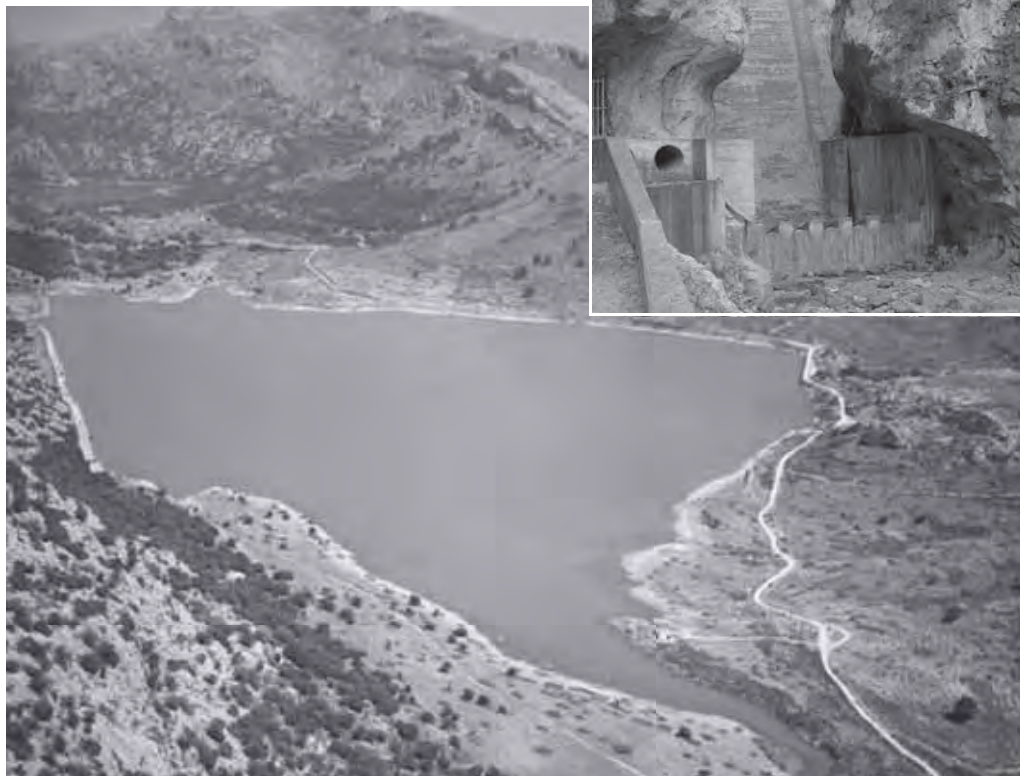
Plate 57. Embalses raw water reservoir of 4.8 million m 3 capacity for water supply of Palma (above), and the reservoir of Gorg Blau of 6.4 million m 3 on the back (Photo: EMAYA)
