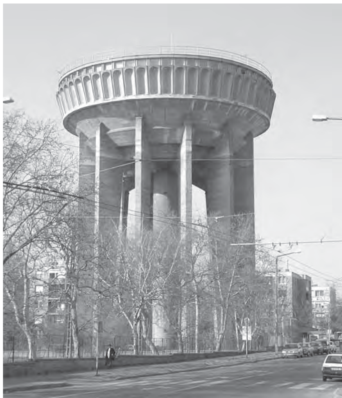
Plate 20. Dobozi housing estate water tower in Debrecen, Hungary (Photo: Victor Pál, 2004)
