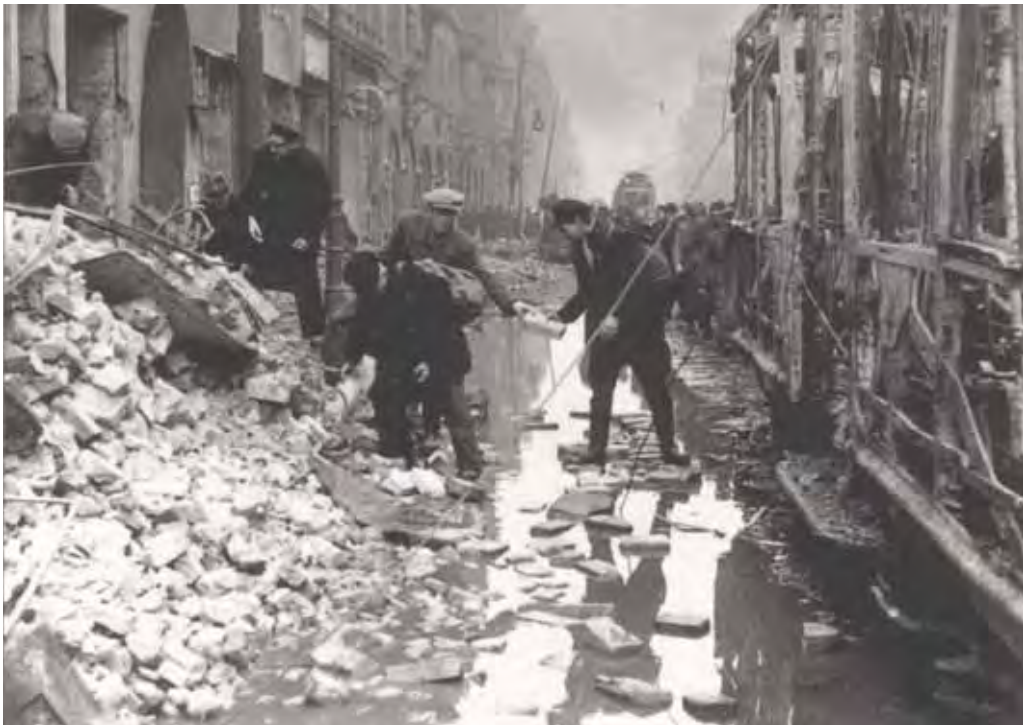
Plate 15. Water main burst after an air raid on 3 January, 1945 in Berlin, Germany at the end of World War II (Photo: Bärthel 1997, 188; with the permission of Berlin Wasser)
