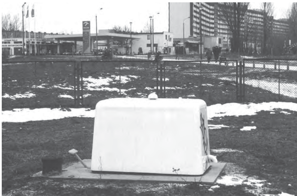
Plate 41. A covered ground water well in Gdańsk, Poland (Photo: Agata Depka, 2004)
