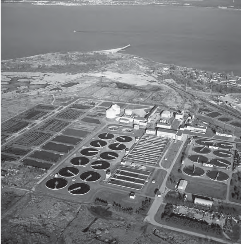
Plate 7. Paljassaare Wastewater Treatment Plant, Tallinn, Estonia (Photo: AS Tallinna Vesi)
