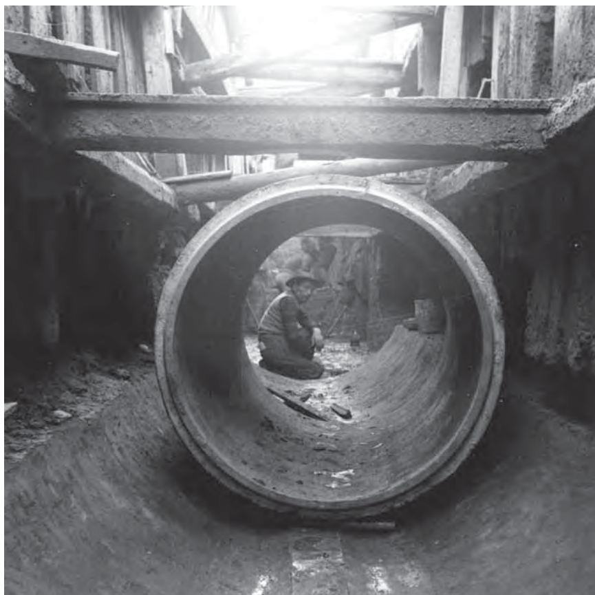
Plate 26. Construction of sewers in Bologna, Italy in the 1930s–1940s (Photo: Hera)
