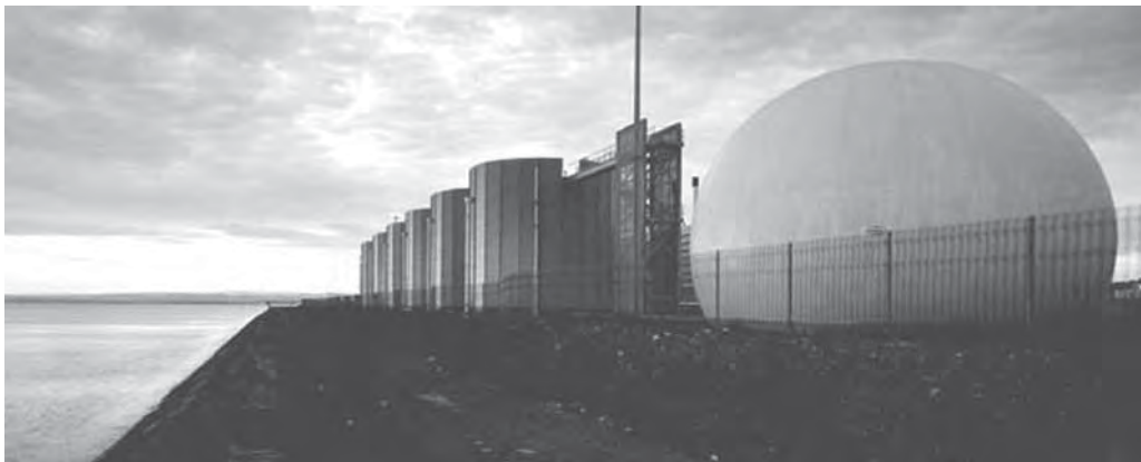
Plate 65. Digestors and gas holders of Sealand wastewater treatment plant in Edinburgh, Scotland, refurbishment completed in 2003 (Photo: Scottish Water)
