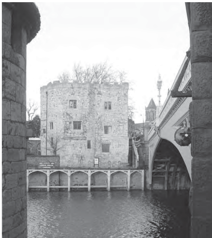
Plate 61. Lendal water tower in Leeds, England, dating back to the 14 th century, in more recent years used as the headquarters of York Waterworks, purchased by Yorkshire Water in 1999 (Photo: Yorkshire Water)
