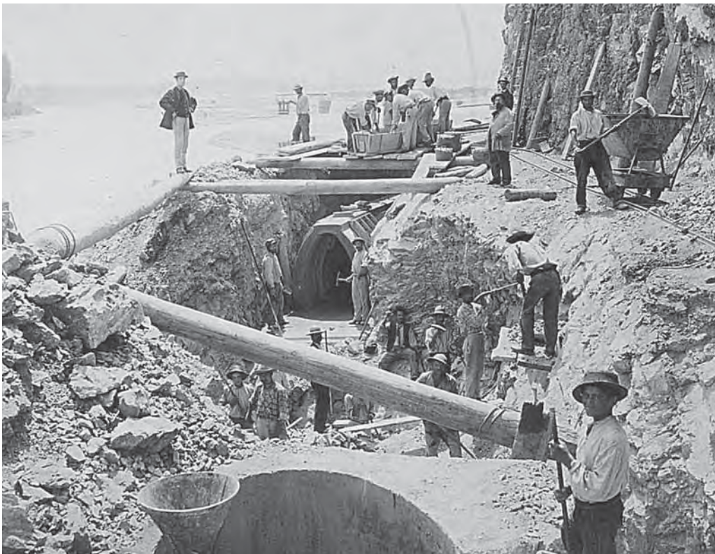
Plate 12. Construction of a drain collector in the late 1800s in Grenoble, France (Photo: Régie des Eaux de Grenoble)
