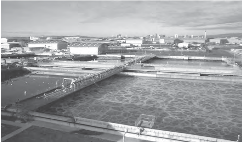
Plate 63. New wastewater treatment plant in Cardiff East, Wales (Photo: Dwr Cymru Welsh Water)
