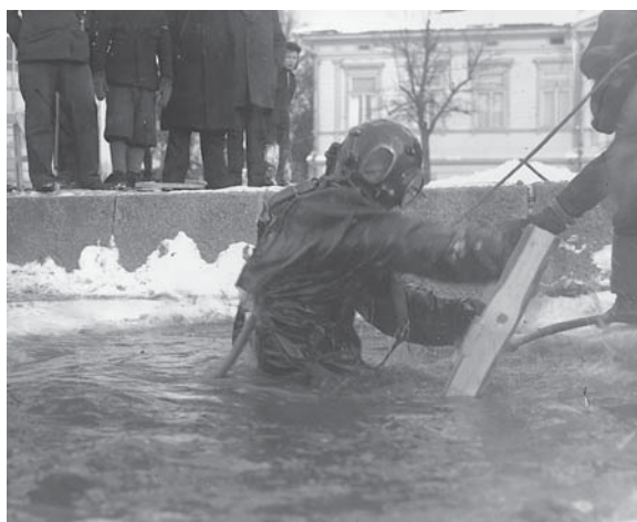
Figure 2 Installation of the watermain under the Porvoo River in 1937. (Porvoo Water)
