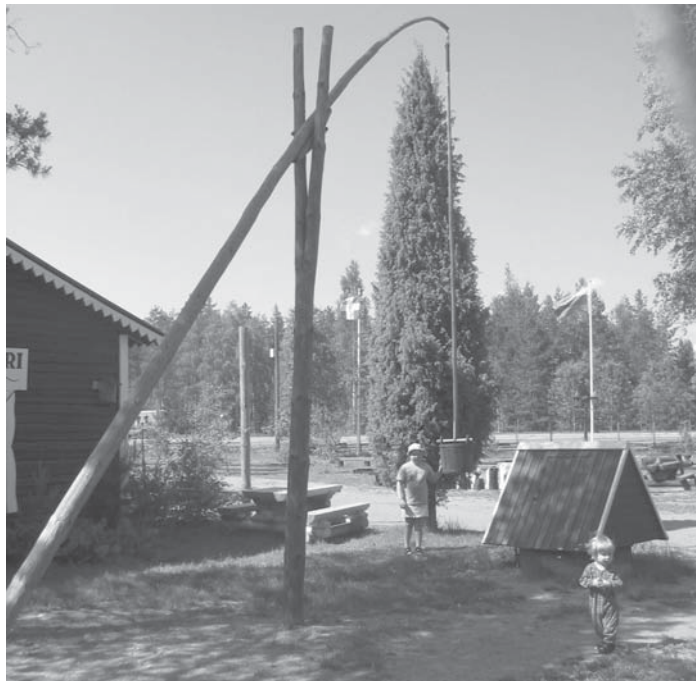
Figure 4 A well with counterpoise lift. (P. Juuti)
