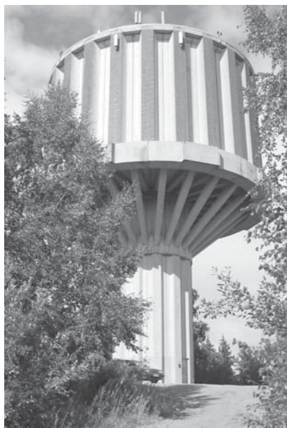
Figure 1 Water tower of Slätberget. It was completed in 1997 and has capacity of 2,000 m 3 . (P.Juuti)
