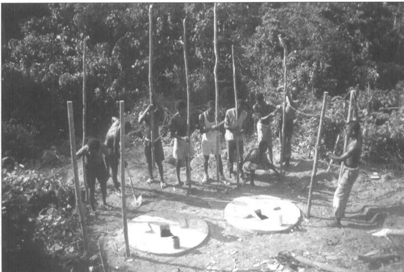
No construction without consultation — sanitation programmes must be planned with full community participation.
