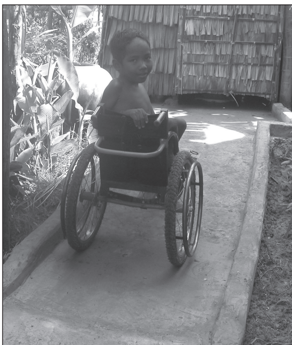
Figure 5.9. Concrete ramp from house to bathing area and toilet.
