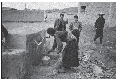
Figure 9.161. Original tapstand, with low taps only. Difficult to use for people with back problems.
