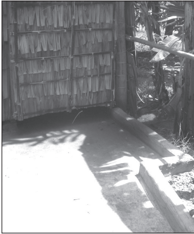
Figure 9.71. Flat platform in front of toilet door.
