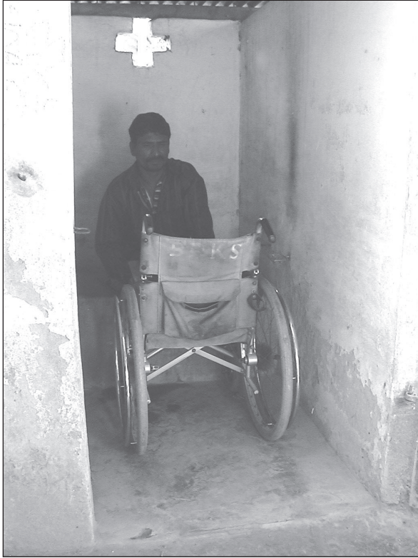
Figure 5.25. Toilet with space for wheelchair user to enter, but not to turn. User must reverse out. (Case-study 9.1, page 154)
