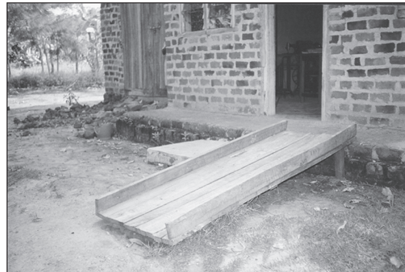
Figure 5.12. Movable wooden ramp.
