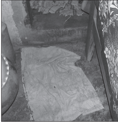
Figure 9.103 Floor cloth at the bathroom door.
