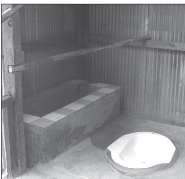
Figure 9.95. Wooden handrail from door to back wall of toilet.
