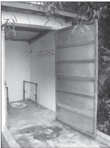
Figure 9.79. Smooth entrance to toilet. Note lack of flat platform in front of door which is a problem.
