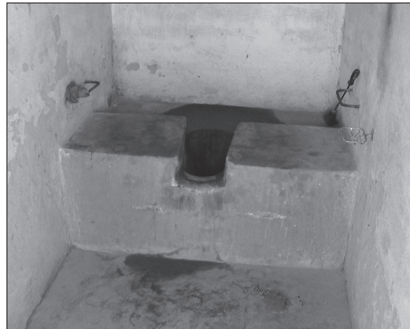
Figure 7.31. Cement-plastered brick platform with commercially available PVC toilet pan inset. Sitting blocks at height for easy wheelchair transfer. (Case-study 9.1, page 154)
