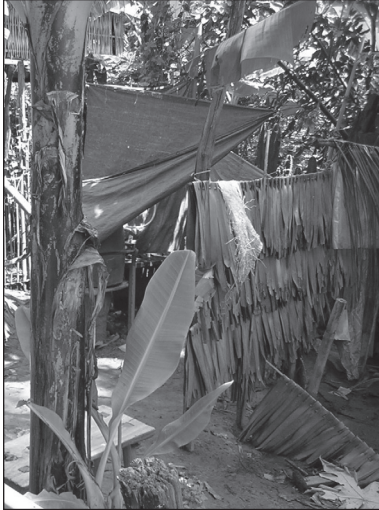
Figure 9.61. Bathing area with leaf screen and plastic sheeting for a door.
