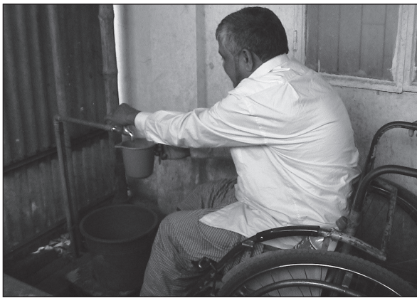
Figure 6.14. A wheelchair user collects water from a tap ~90cm high. (Case-study 9.3, page 164)
