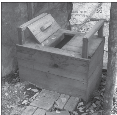
Figure 9.89. Wooden toilet seat showing the lid removed from the toilet hole.
