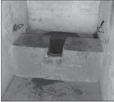
Figure 9.4. Raised brick toilet platform with inset PVC pan.
