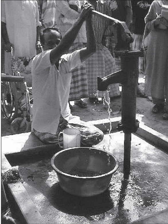
Figure 6.3. Low concrete sitting platform built into pump apron. (Case-study 9.2, page 161)
