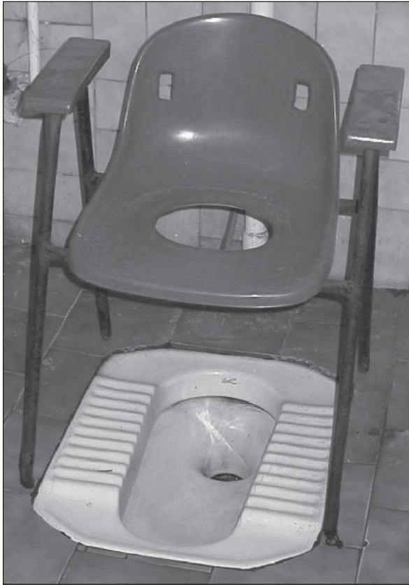
Figure 7.34. Moulded plastic toilet seat: durable, easy to clean, hygienic. High cost. Hole quite far back in seat. No splash-guard.
