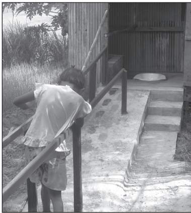
Figure 9.94. Horizontal parallel bars enable child to walk from house to toilet with minimal help
