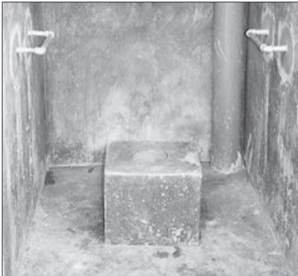
Figure 7.3. Handrails cemented to each side wall of toilet cubicle. H: ~ 80cm – likely to be too high and too far apart for some child users. (Case-study 9.29, page 242)
