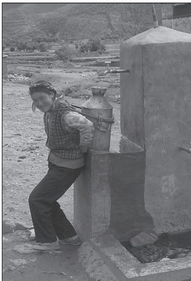
Figure 9.160. 'Back-happy' tapstand in use. Note direction of water drainage into ground-level splash apron.
