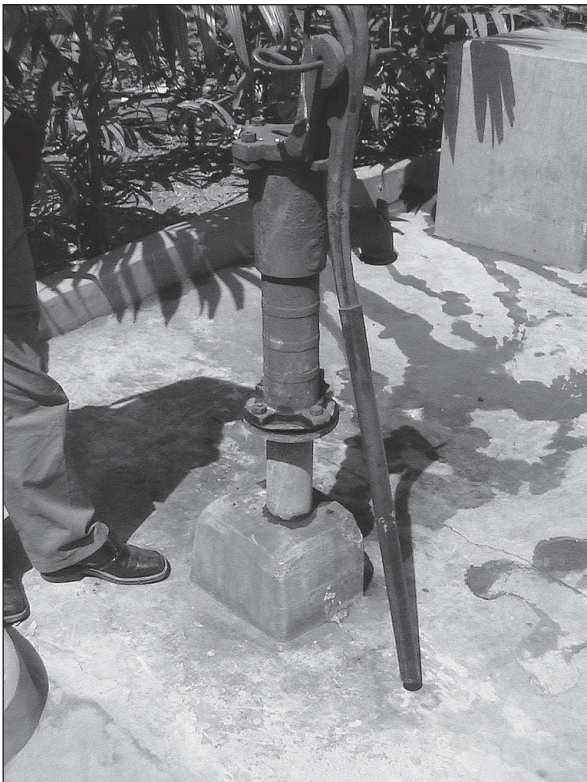
Figure 6.4. Handpump with apron showing direction of water drainage away from pump. Note lengthened handle for extra leverage. (Case-study 9.3, page 164)
