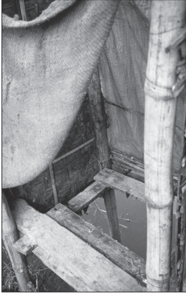
Figure 2.8. Hanging latrine in Bangladesh – a challenge for all but the very agile.
