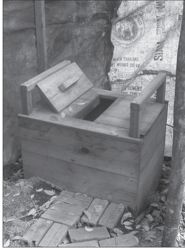
Figure 7.29. Wooden box toilet seat installed over a pit latrine. A cover prevents flies and smells when the toilet is not in use. (Case-study 9.17, page 209)
