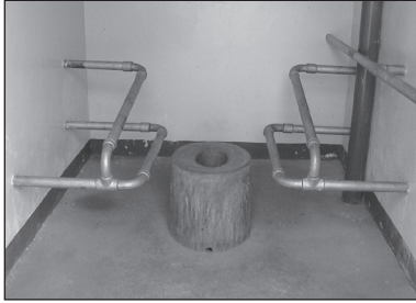
Figure 9.124. Raised toilet seat with handrails for support.
