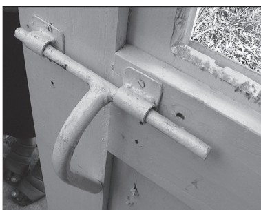
Figure 9.123. Large slide bolt for easy grip.
