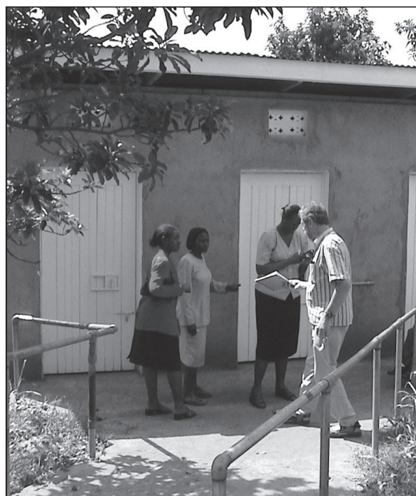
Figure 5.10. Wide concrete ramp with handrails both sides.
