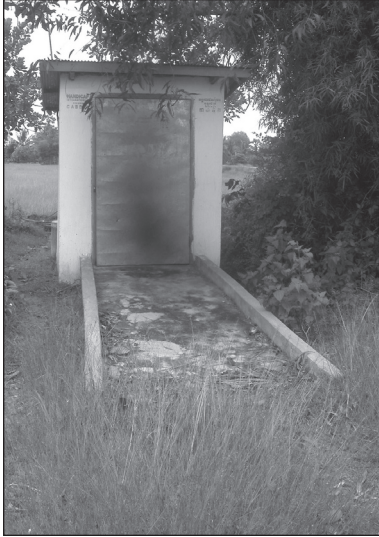
Figure 9.78. The access ramp to the toilet with long grass in the way.
