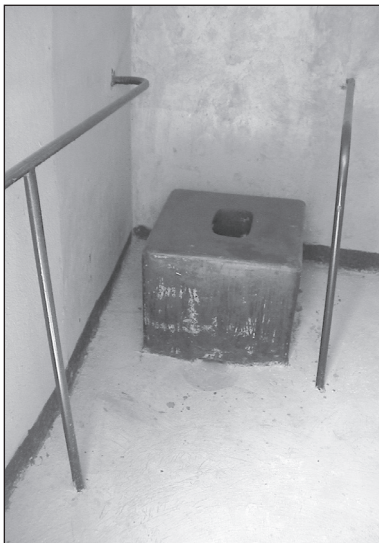
Figure 9.119. Painted cement screed brick toilet seat with handrail on the left from the door.
