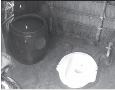
Figure 9.73. Water jar next to toilet pan. Note moulded cement mortar shapes for correct wheelchair positioning.
