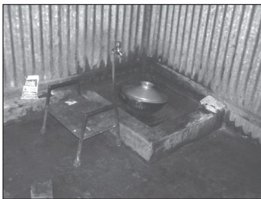
Figure 9.26. Floor level washing up sink with low concrete wall.
