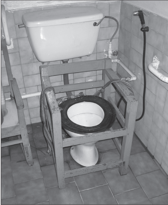
Figure 7.12. Painted wooden frame around pedestal toilet seat.
