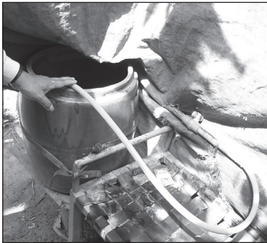
Figure 9.63. Hose with a tap for filling water storage jar.
