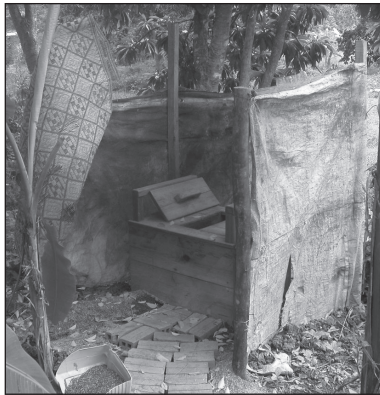
Figure 9.88. Family latrine behind house accessed via brick path. Woven mat used as a door.
