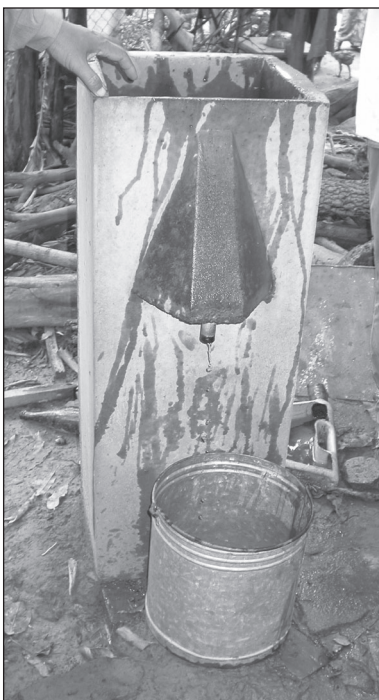
Figure 9.59. Sand water filter.
