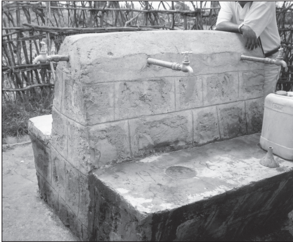
Figure 6.19. Tapstand in Ethiopia. Note the indentation in the shelf to sit round-bottomed containers in while they are filled.
