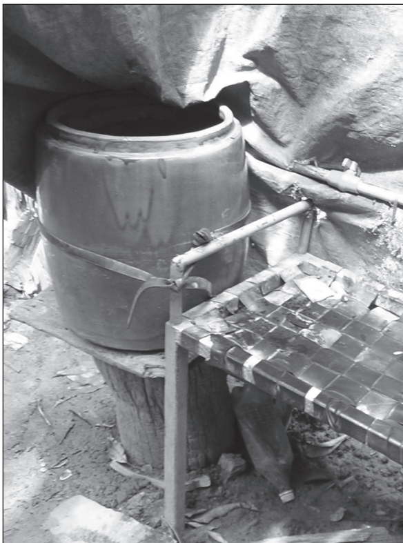
Figure 6.39. Water storage jar in bathing area, raised on a wooden stand and held in place with a rubber strap. (Case-study 9.14, page 197)
