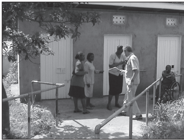
Figure 9.122. Concrete ramp to latrine block with handrail both sides.
