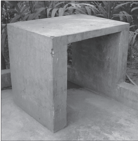
Figure 6.83. Concrete slab for washing clothes. (Case-study 9.3, page 166)
