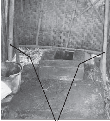
Figure 9.44. Vertical bamboo support poles one on each side of the concrete slab. (CRP)
