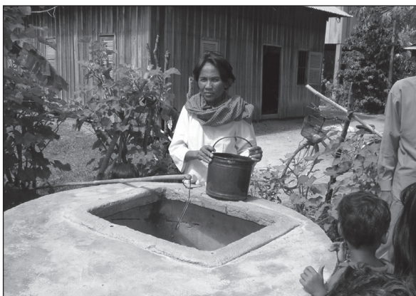
Figure 6.12. A concrete slab cover over the well provides a surface to rest a container.
