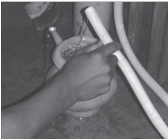
Figure 6.23. A flexible hose attached to a tap allows water to be poured into a container with one hand. (Case-study 9.6, page 177)
