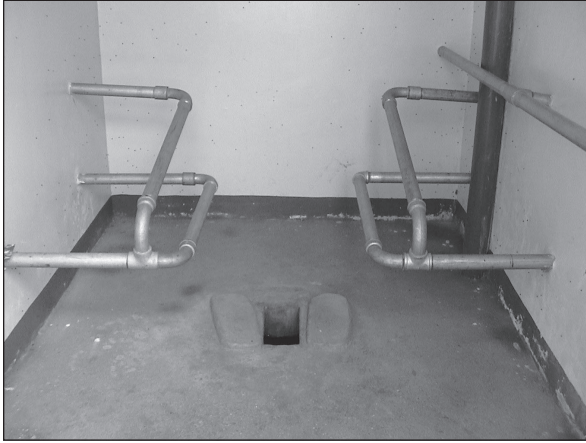
Figure 7.4. Diagonal and horizontal rails fixed to side walls at different heights. Note additional horizontal rail from front to back of wall on the right.
