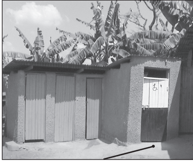
Figure 9.117. Wheelchair accessible toilet on the right. Arrow shows concrete ramp.
