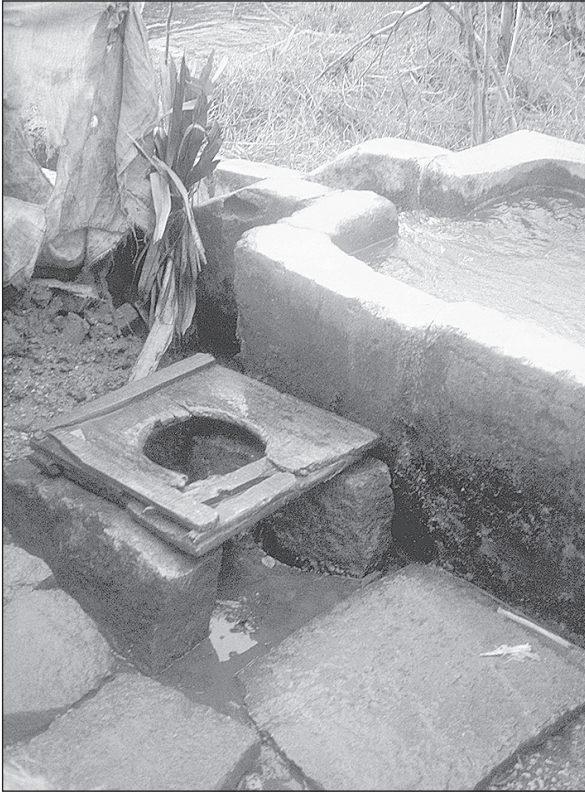
Figure 7.28. Wooden toilet seat supported on two brick blocks over a pit latrine. The pit was dug more than 2m deep to avoid contaminating the water source. Location next to the water trough makes water for anal cleansing and handwashing easily accessible.
