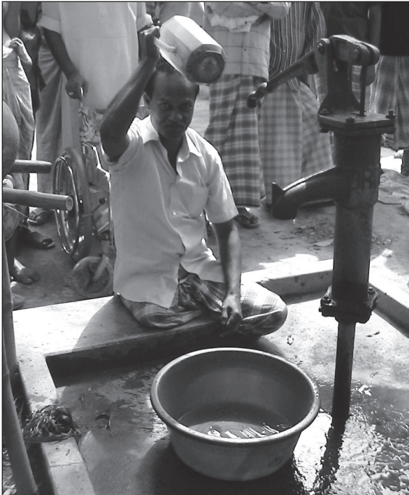
Figure 6.48. Low concrete sitting platform. (Case-study 9.2, page 161)
