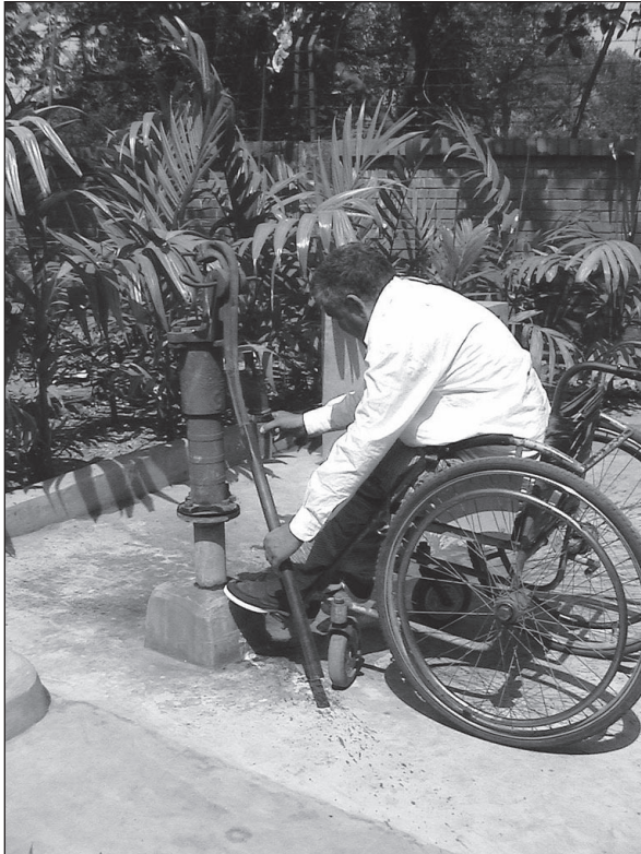
Figure 6.5. The same handpump operated by a wheelchair user on a level apron. (Case-study 9.3, page164)
