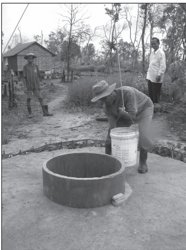
Figure 9.50. Lifting the bucket over the well wall.
