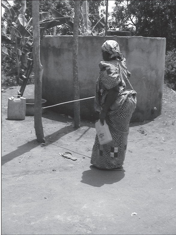
Figure 5.13. Two fixed wooden posts act as landmarks for a blind woman to find her way to and from the water tank or toilet. For a user with some vision, posts could be painted/marked a bright colour.
