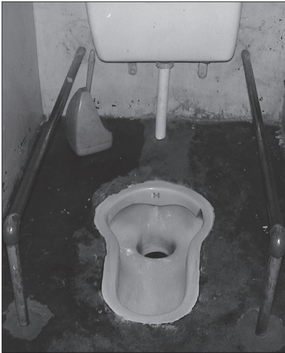
Figure 7.1. Handrail attached to floor on both sides of a squat toilet. H: ~30cm. (The wide toilet pan is not recommended.)
