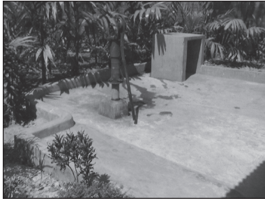
Figure 9.13. Handpump with wide concrete apron for easy wheelchair access on three sides.
