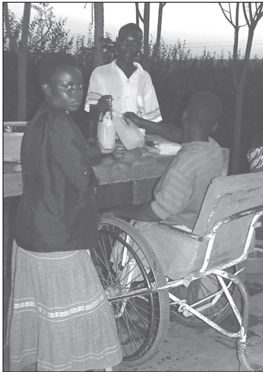
Figure 9.97. Knee-hole under concrete shelf allows wheelchair user to get close to reach tap.
