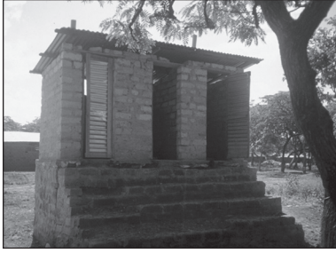
Figure 2.4. Latrine in Tanzania with steep steps and narrow doors.
