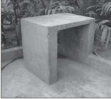
Figure 9.16. Concrete laundry slab located on edge of handpump apron.
