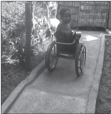
Figure 9.68. Concrete ramp leading to bathing area.
