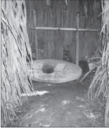
Figure 9.45. Bamboo support rail.
