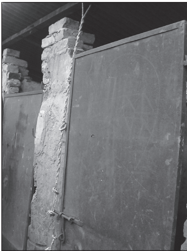
Figure 9.40. Rope hanging from roof beam.
