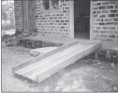
Figure 9.149. Movable wooden ramp.
