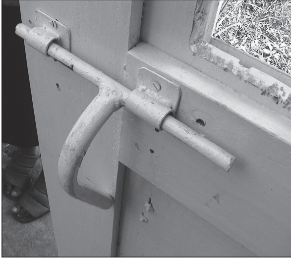
Figure 5.23. Large bolt, easy to grasp. The small window allows the door to be opened from outside.
