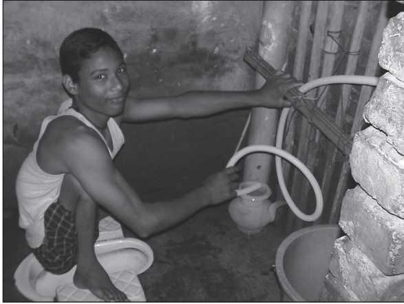
Figure 7.8. Horizontal wooden bar tied to existing pipes in front of toilet. H of bar (~70cm) was decided by user. No choice of distance for bar – nearer would be more comfortable. (Case-study 9.6, page 177)
