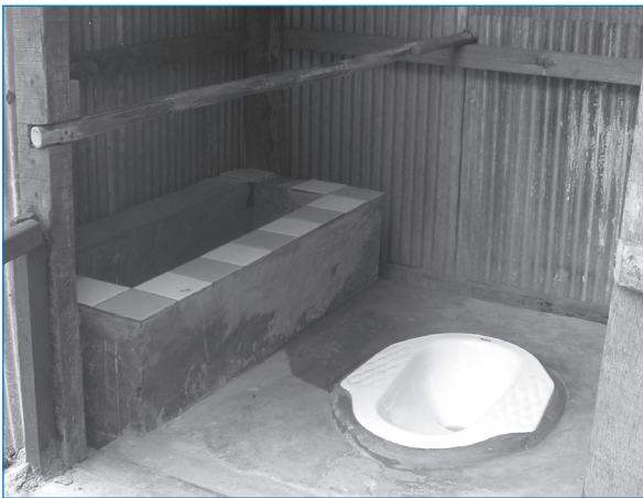
Figure 6.41. Water trough next to the toilet. (Case-study 9.19, page 215)
