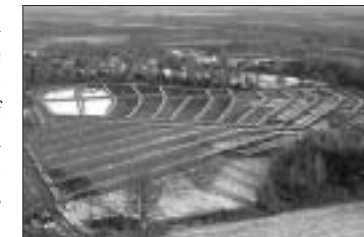
Specially designed mud storage lagoons
