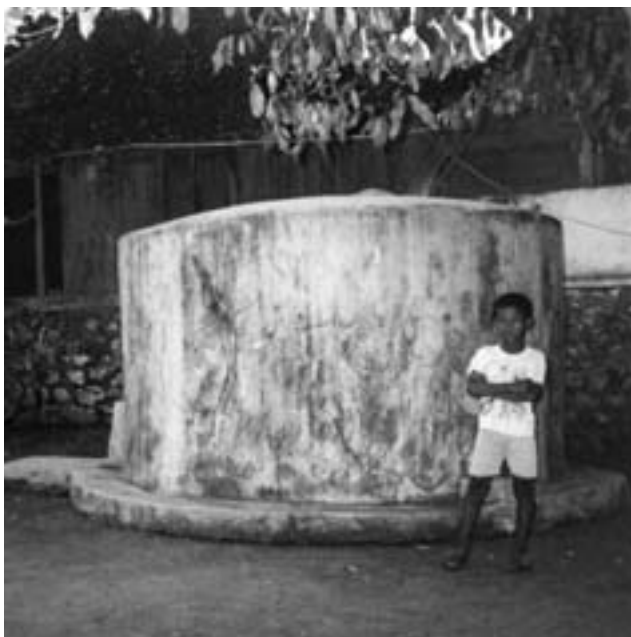
Closed rainwater storage tank
