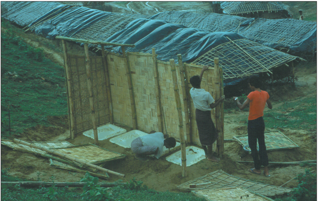
Borehole latrines nearing completion, Bangladesh
