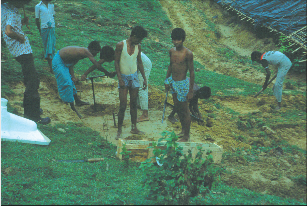
Drilling boreholes for latrines, Bangladesh
