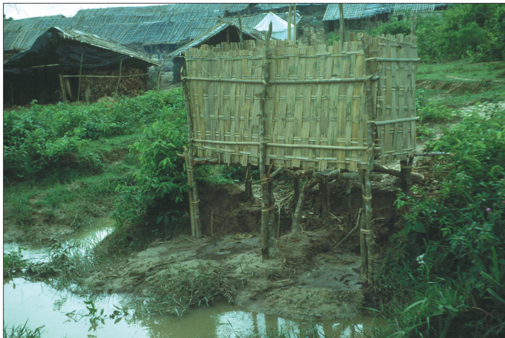
Overhung latrine, Bangladesh
