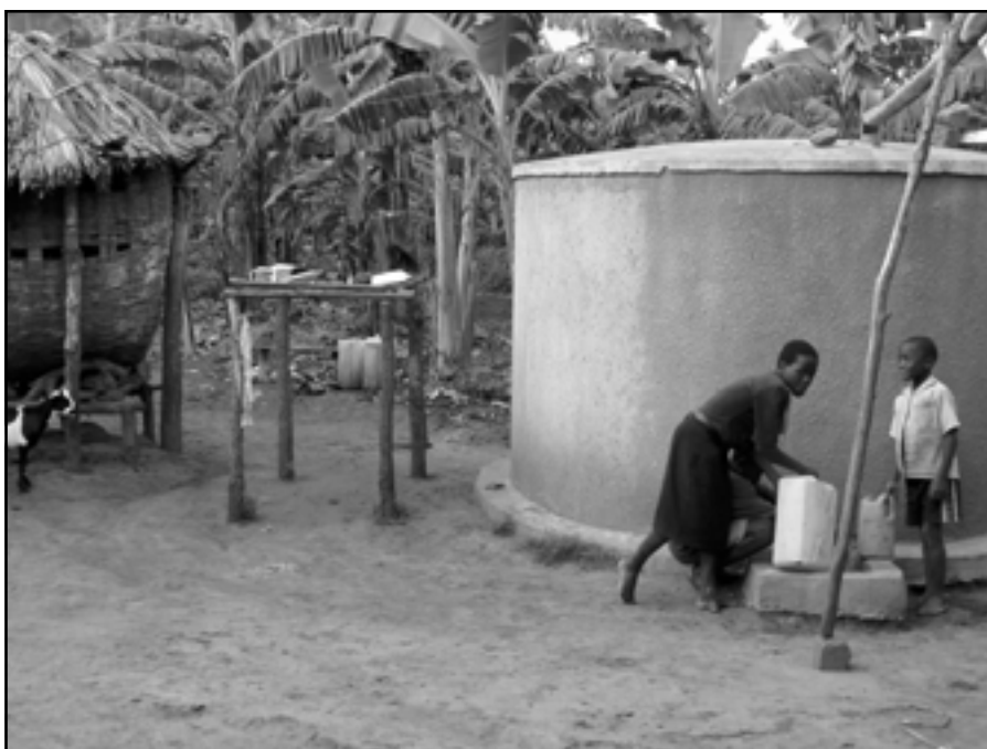
This rainwater tank in Uganda has a capacity of 10 m 3 and is made of ferrocement
