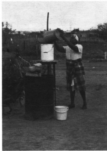
Using the iron removal plant: note tubewell behind to the right.
