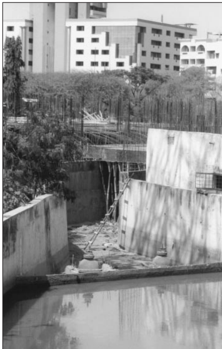
This multi-storeyed building is being constructed on a storm drain
