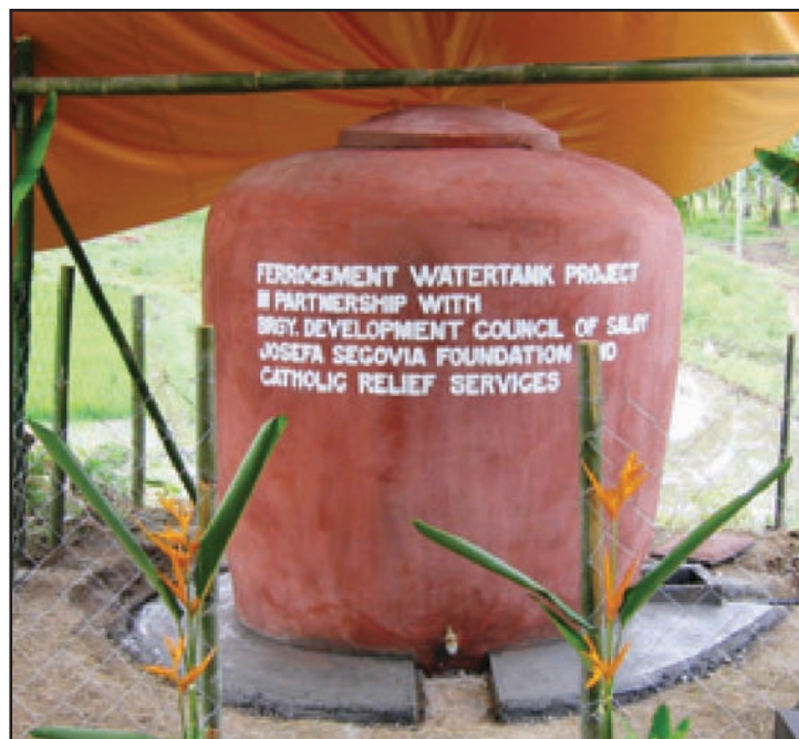
Fig. 73: Completed Tank with lid, valve box and optional splash-pad for erosion prevention
