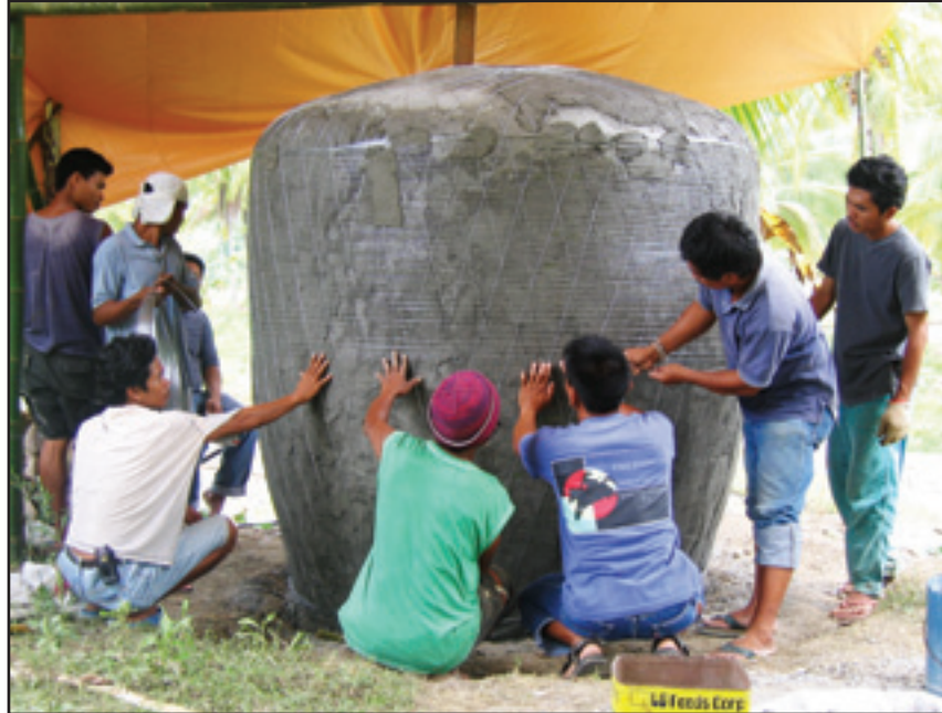
Fig. 66: Horizontal wire reinforcement
