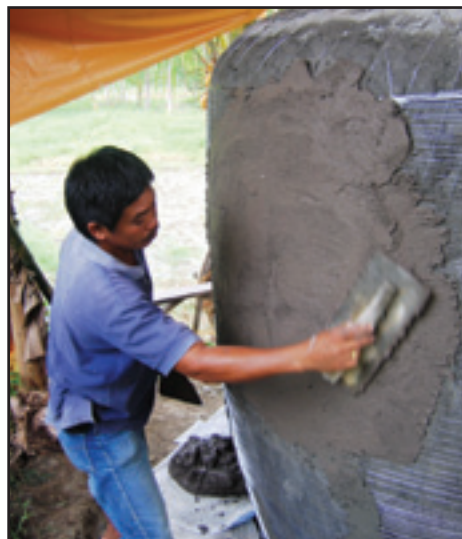
Fig. 67: Applying the final layer
