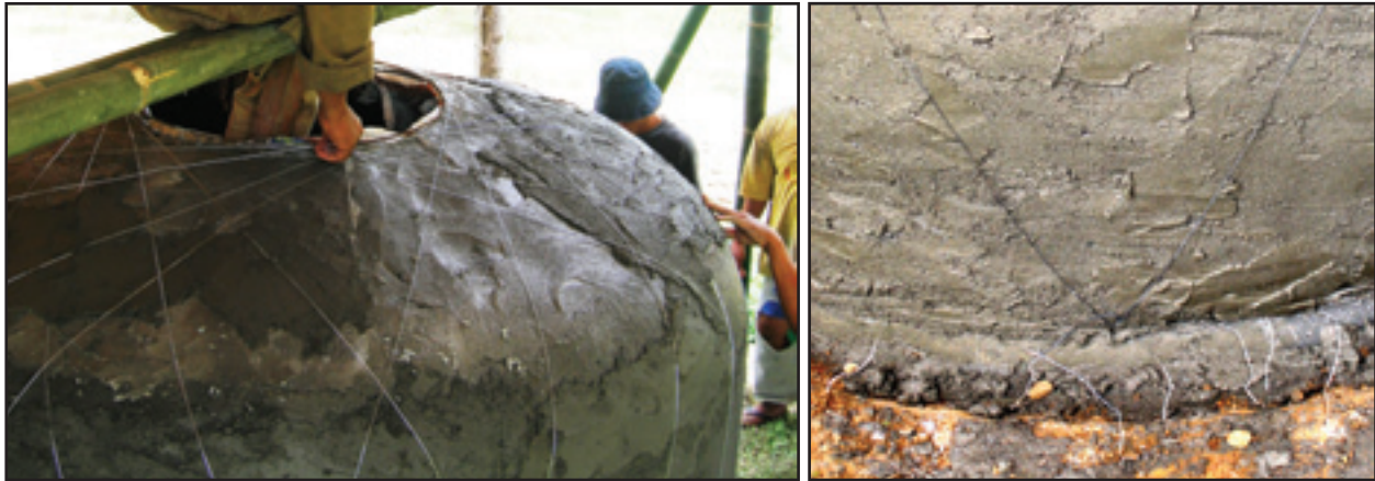
Figs. 61–62: Wire placement in relation to the rim, and Connecting the wire to the tank base
