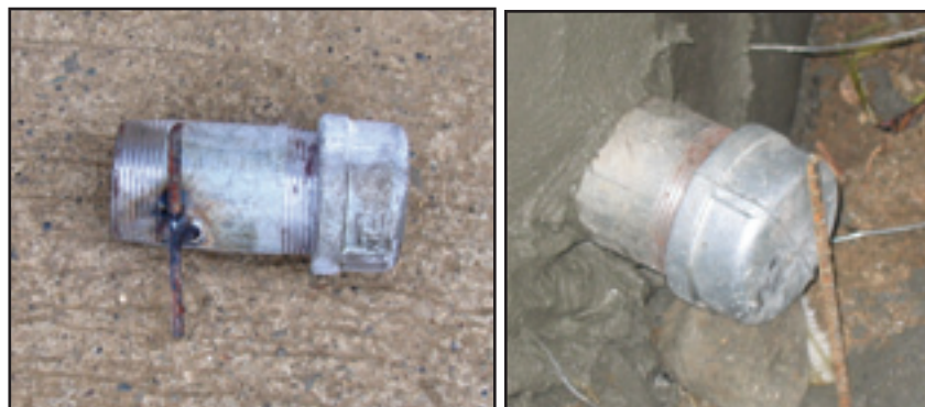
Figs. 58–59: Attaching pipe fittings
