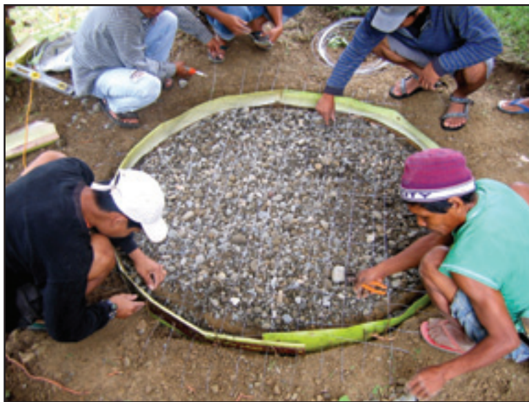
Fig. 51: Adding base reinforcement
