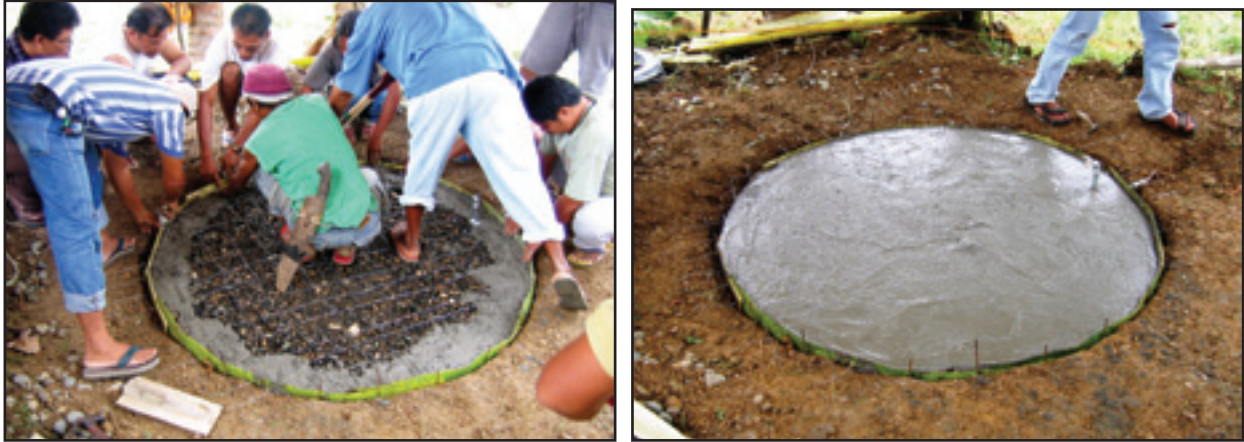
Figs. 52-53: Pouring cement and The completed base
