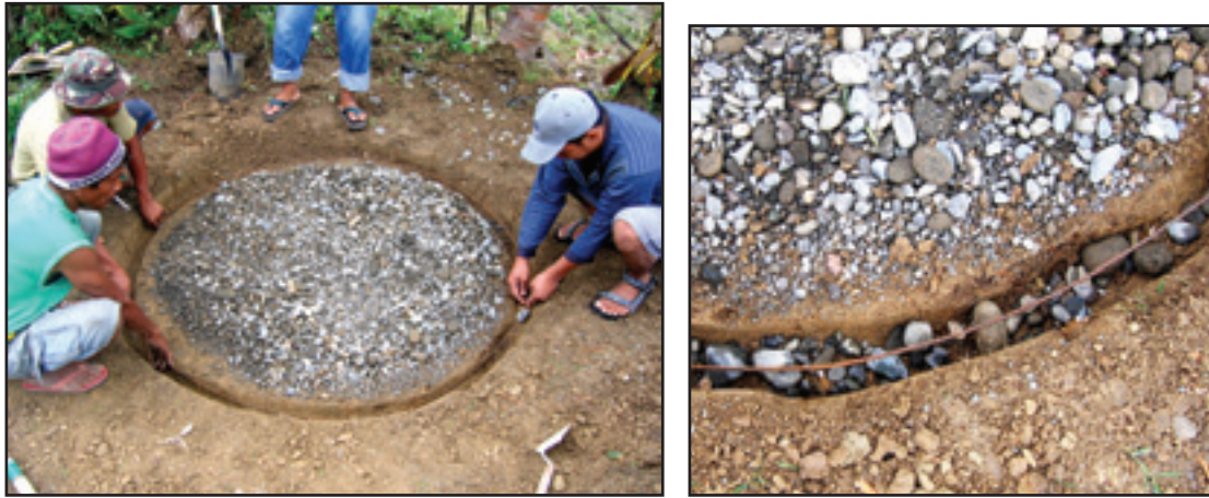
Fig. 49-50: Excavating the base and Adding gravel
