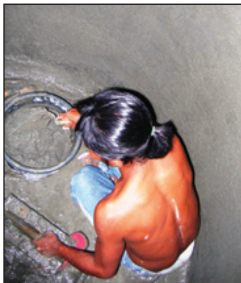
Fig. 71: Plastering the inside of the tank
