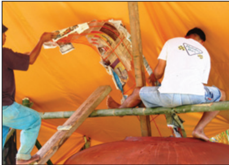
Fig. 70: Removing the form
