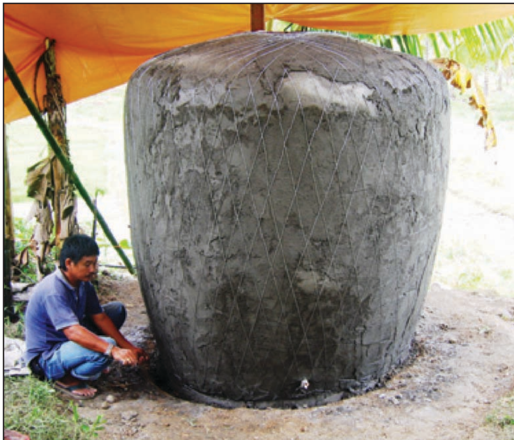
Fig. 63: Completed vertical wire reinforcement
