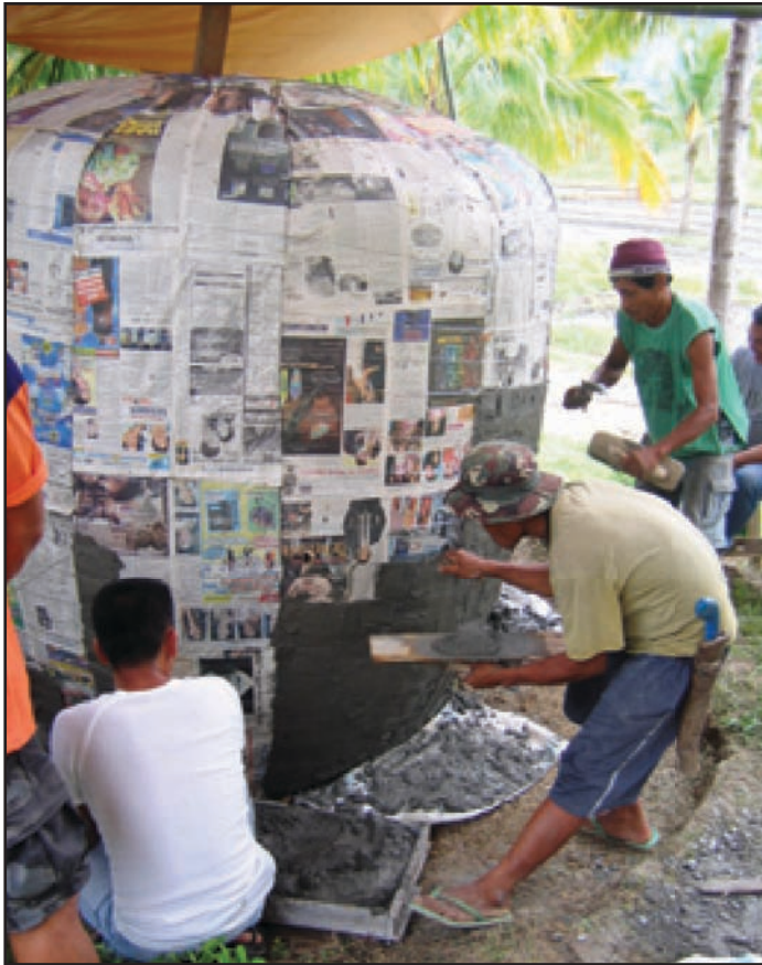
Fig. 57: Plastering the first layer
