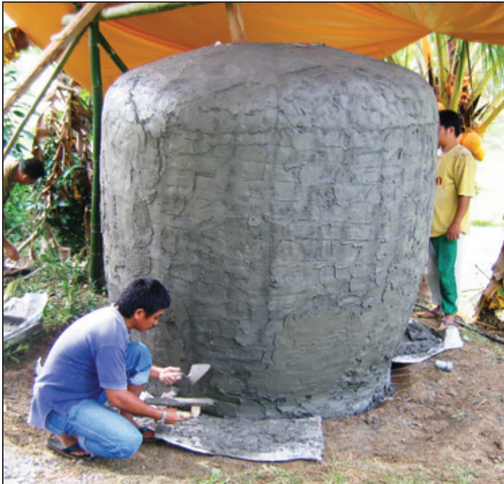
Fig. 60: Plastering the second layer
