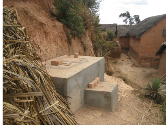
Figure 4: Unfinished type III latrines
