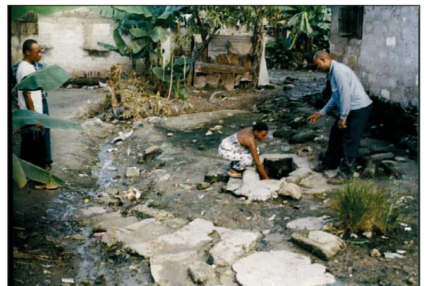
Shallow water well. Looking on is the village Chairperson and one of the Community Assessment Team members, Dar-es-Salaam, Tanzania.
