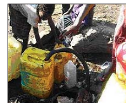
One of the public taps whose pipes have been removed and a garden hose attached.
