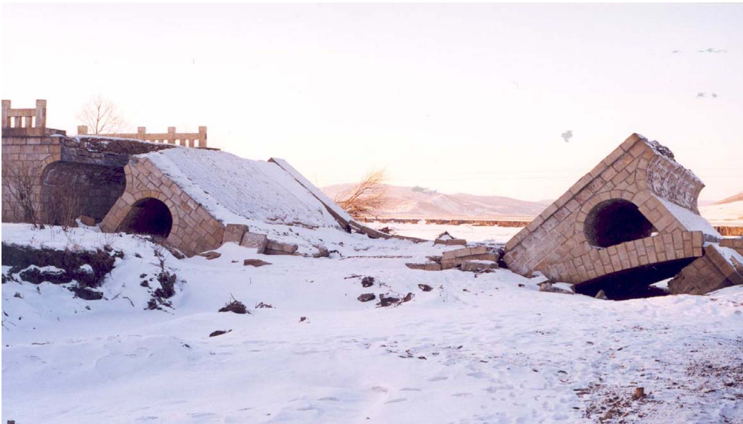
Bridge destroyed by flash flood in Inner Mongolia (1998)
