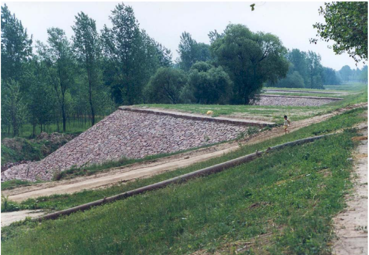
Protective spurs along the Yellow River flood control embankment (1999)
