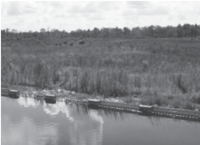
Figure 3-19. Orange County, Florida, Redistribution Constructed Wetland
