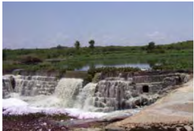
Hyderabad, India – wastewater being diverted over weir into irrigation canals. Source: International Water Management Institute
