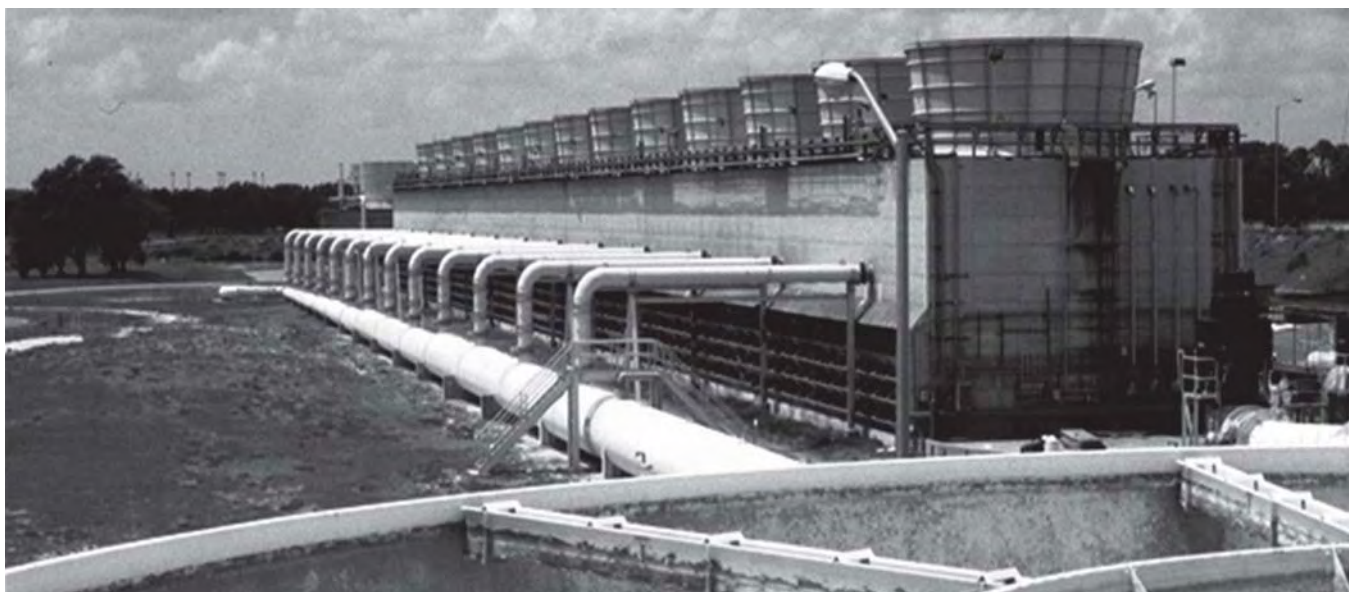
Figure 2-3. Cooling Tower
