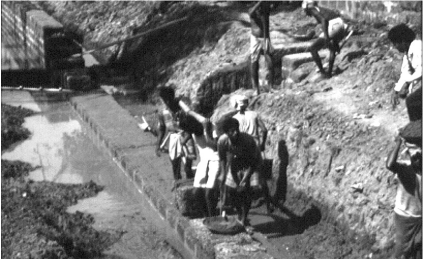
Photograph 2: Micro contractors improving secondary drainage, Cuttack, India
