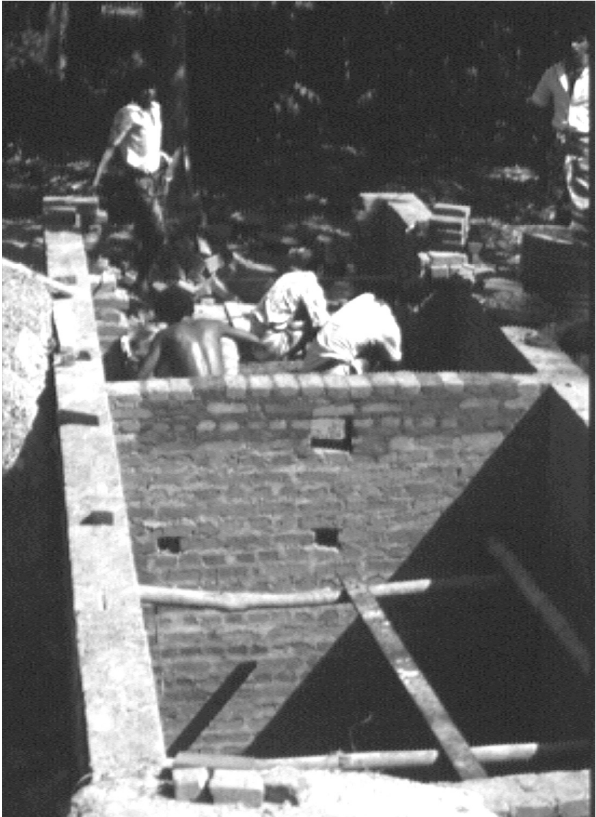
Photograph 1: Septic tank construction by community contractor in Colombo, Sri Lanka
