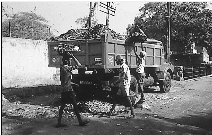
Truck with loading height of around 2 metres; waste is falling onto the loader's head.
