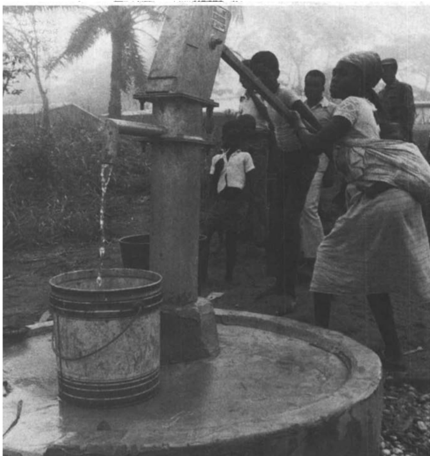
The Decade has succeeded in introducing low-cost appropriate technologies, like this UNICEF-developed India Mark II handpump.
