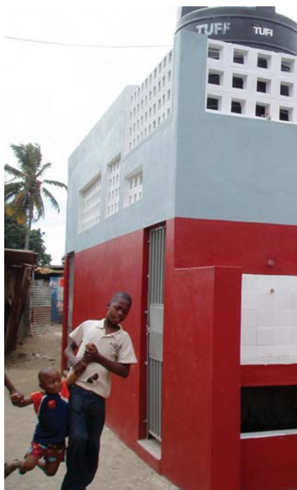
Tchemulane communal facility
