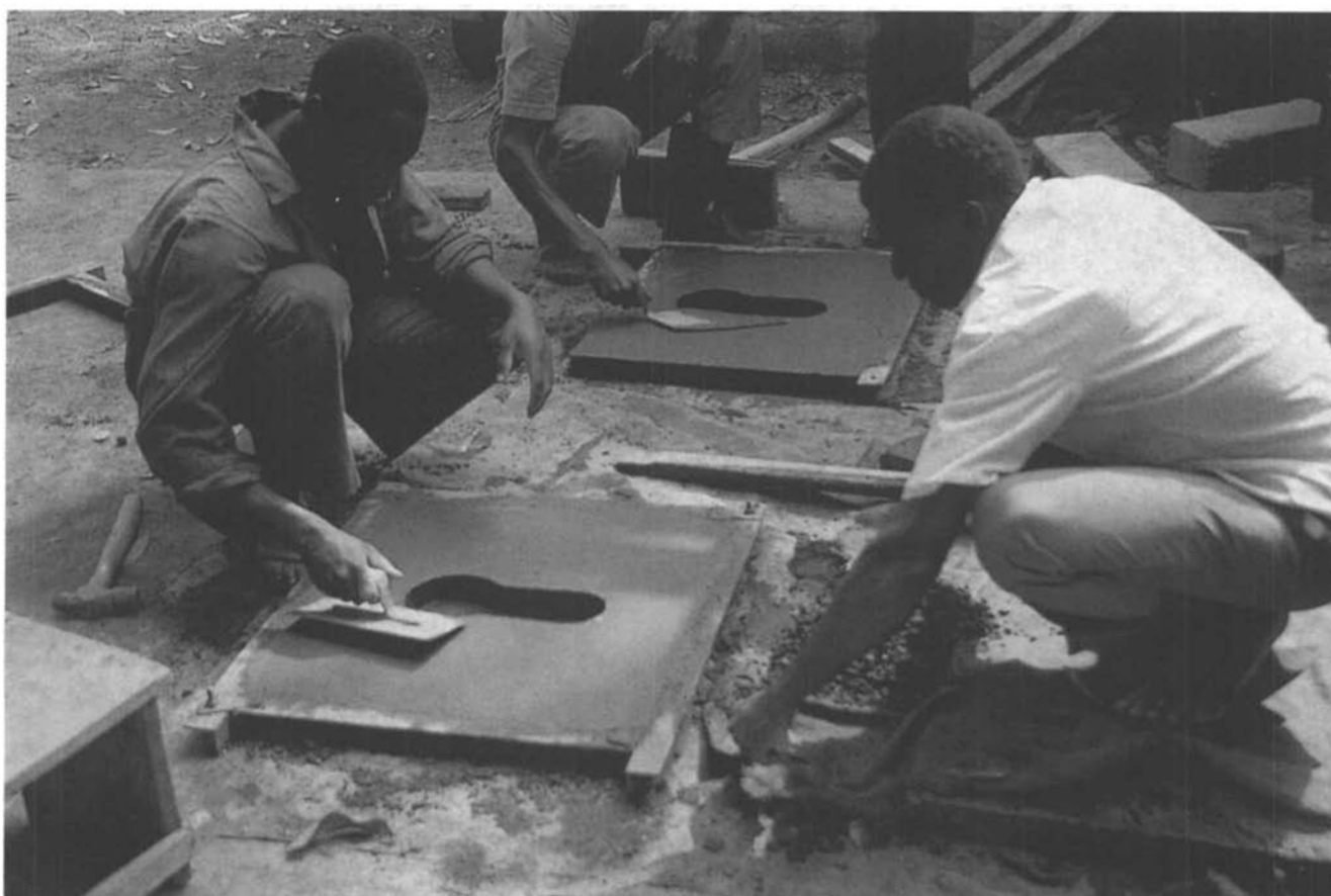
Trainee fundis learning to cast sanplats with keyhole-shaped drop holes.
