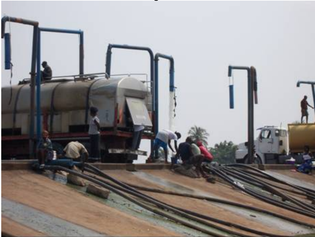
Photo 1: Tanker-trucks filling up from River Bengo at the ANGOMENHA Girafas at Kifongondo 10
