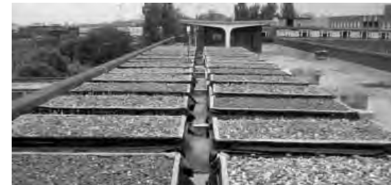
Figure 2.7.2a Brown roof installation trays at the University of Birmingham
