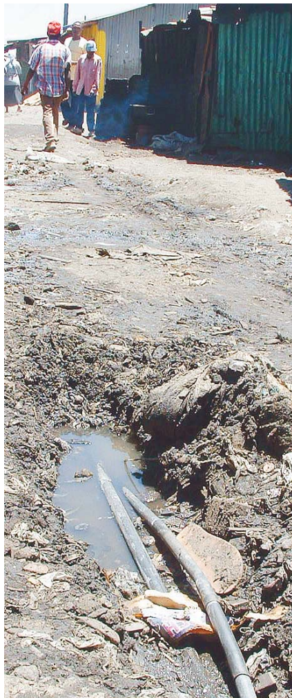
Pipes supplying water kiosks find their way through sludge and solid waste
