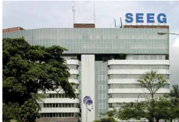
SEEG, the national private operator in Gabon, manages small rural schemes.
