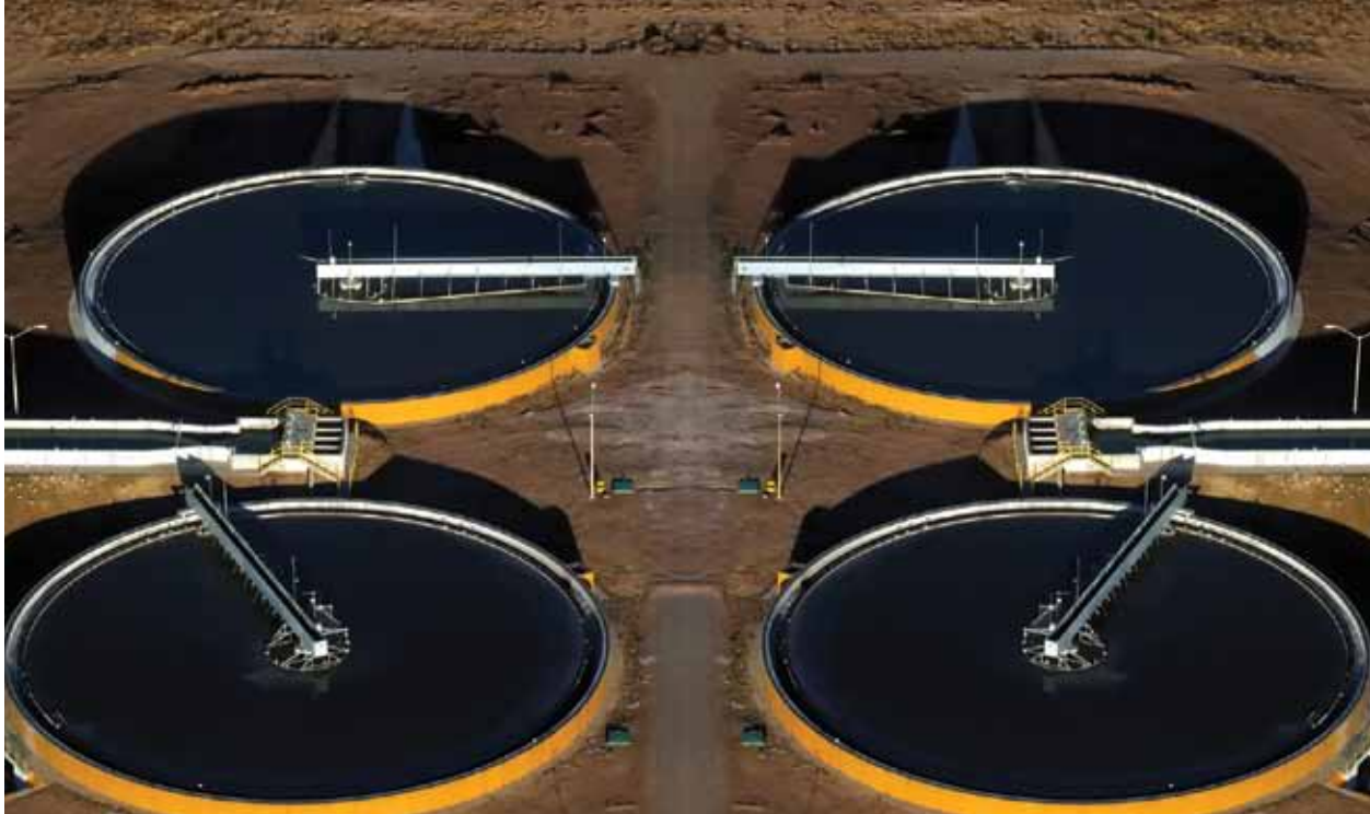
Wastewater treatment plant.
