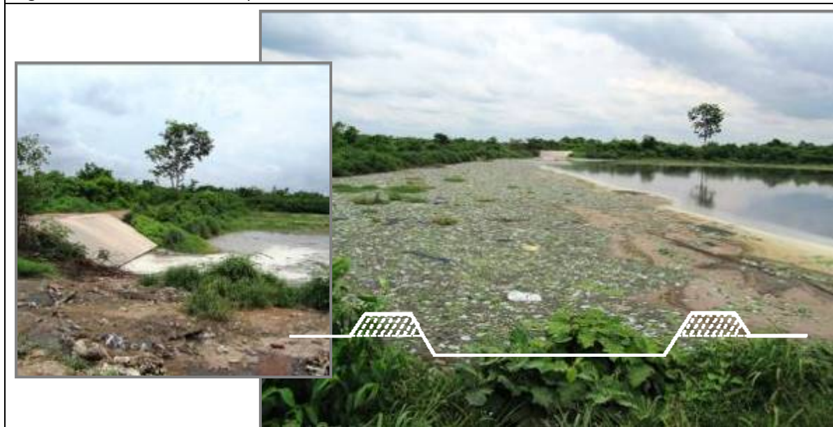
Figure 4.3: Waste stabilisation pond at KM32
