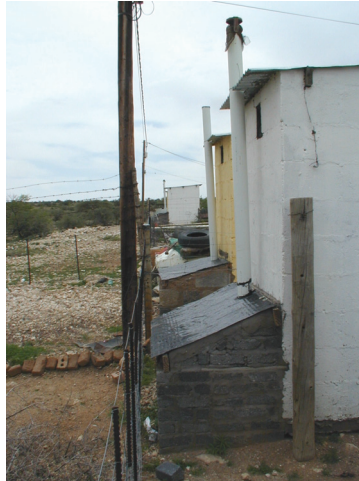
Figure 2.16: Conversion of bucket toilets in Campbell, Northern Cape (Photograph: R. Holden, Mvula Trust)
