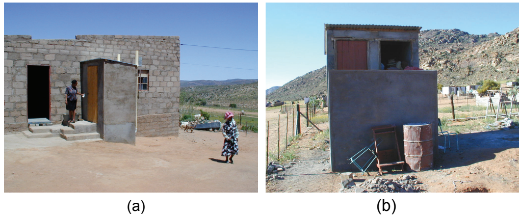
Figure 2.14: Double chamber urine-diversion toilets in Spoegrivier, Northern Cape. (a) Toilet added onto house; (b) separate toilet structure.
