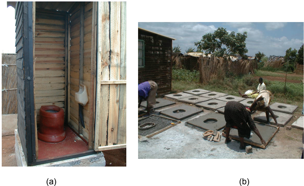
Figure 2.11: Urine-diversion toilets in Zimbabwe.
