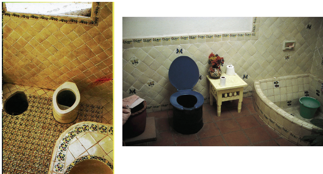
Figure 2.5: The Mexican version of the Vietnamese double-vault toilet, installed in the bathrooms of modern houses in the city of Cuernavaca. The toilets have movable urine-diversion pedestals. The processing chambers below the bathroom floor are accessible from outside the house (César AZorve, CITA, A.C., Mexico)
