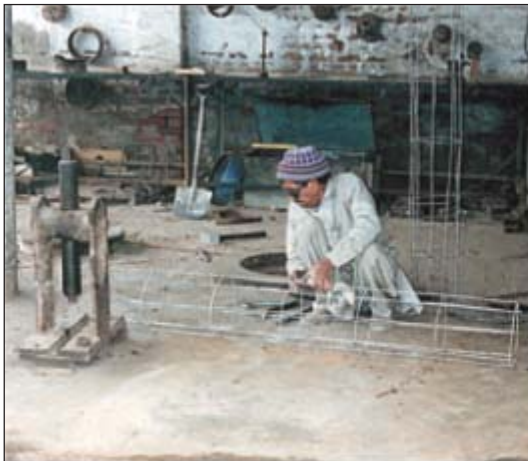
Figure 2-1 Welding the reinforcement cage
