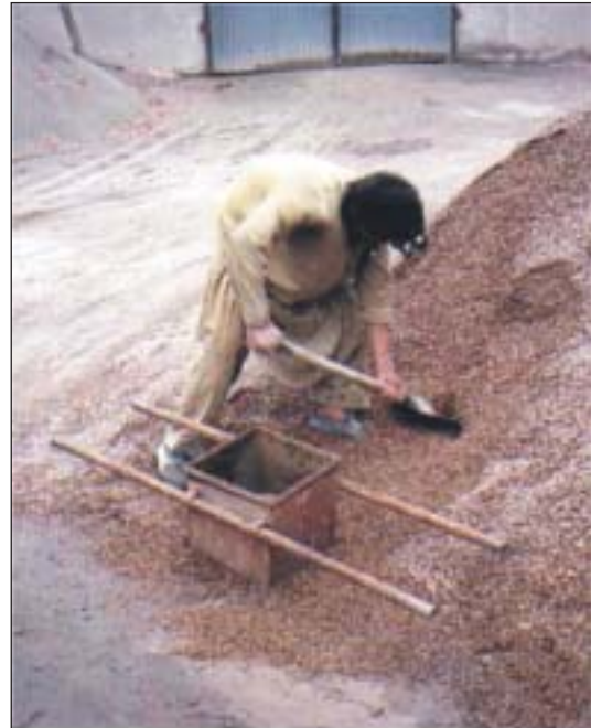
Figure 3-7 Measuring cement using a standard sized container
