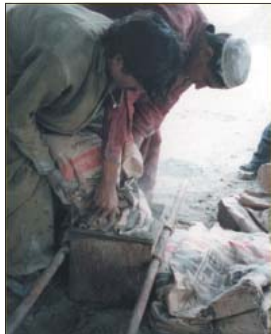
Figure 3-7 Measuring cement using a standard sized container
