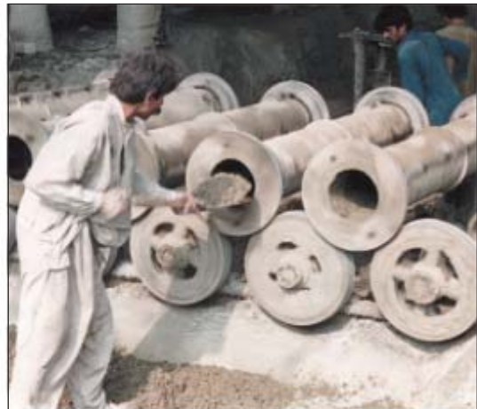
Figure 2-3 Placing concrete in spinning moulds
