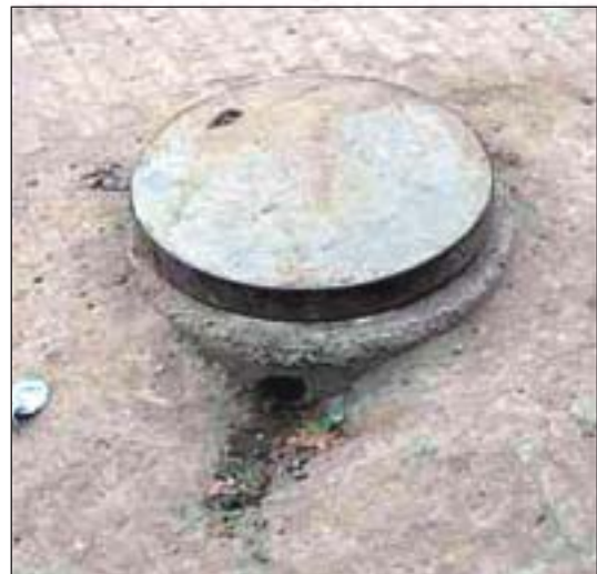
Figure 2-11 Modifications to the manhole cover to drain surface water
