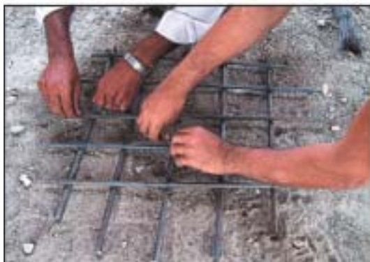
Figure 2-13 Arrangement of the cover reinforcement bars
