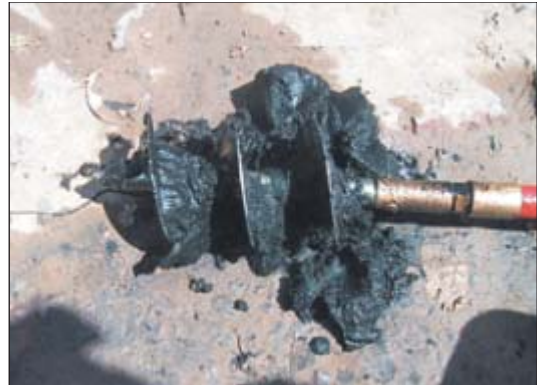
Figure 4-6 Compacted silt removed using the auger borer
