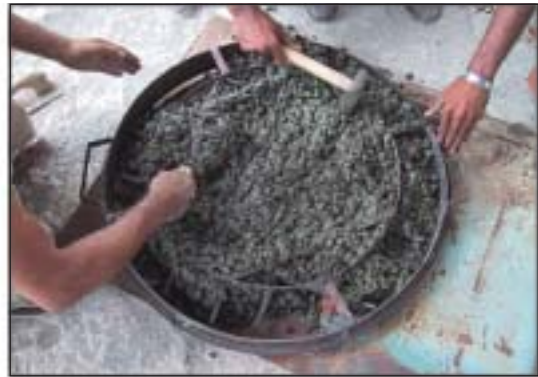
Figure 2-15 Access cover before curing
