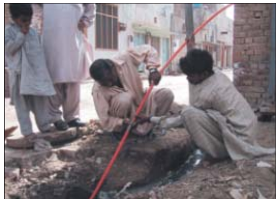
Figure 4-7 Inserting the rodding into the access chamber
