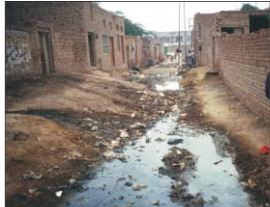
Figure 1-1 Typical sanitation problems associated with poor drainage
