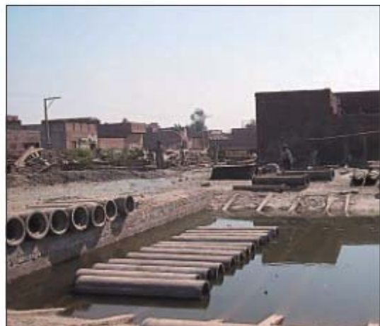
Figure 2-4 Curing the pipes
