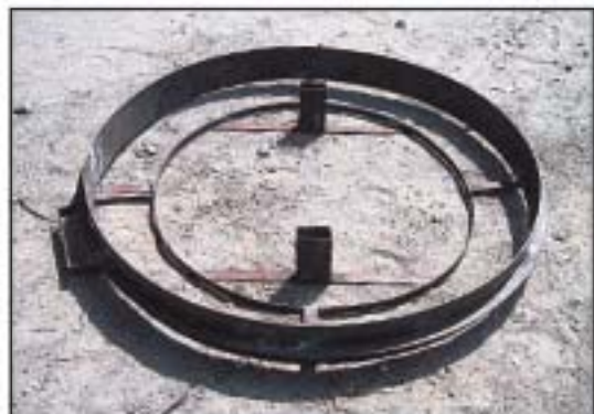
Figure 2-15 Access cover before curing
