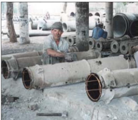
Figure 2-2 Assembling the moulds
