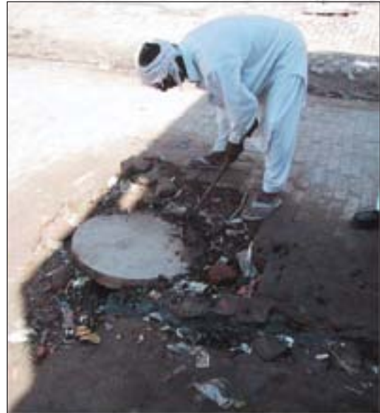
Figure 2-11 Modifications to the manhole cover to drain surface water
