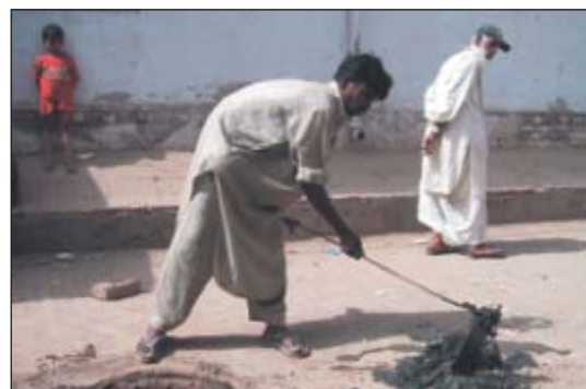
Figure 4-10 Sewer cleanings emptied on the street
