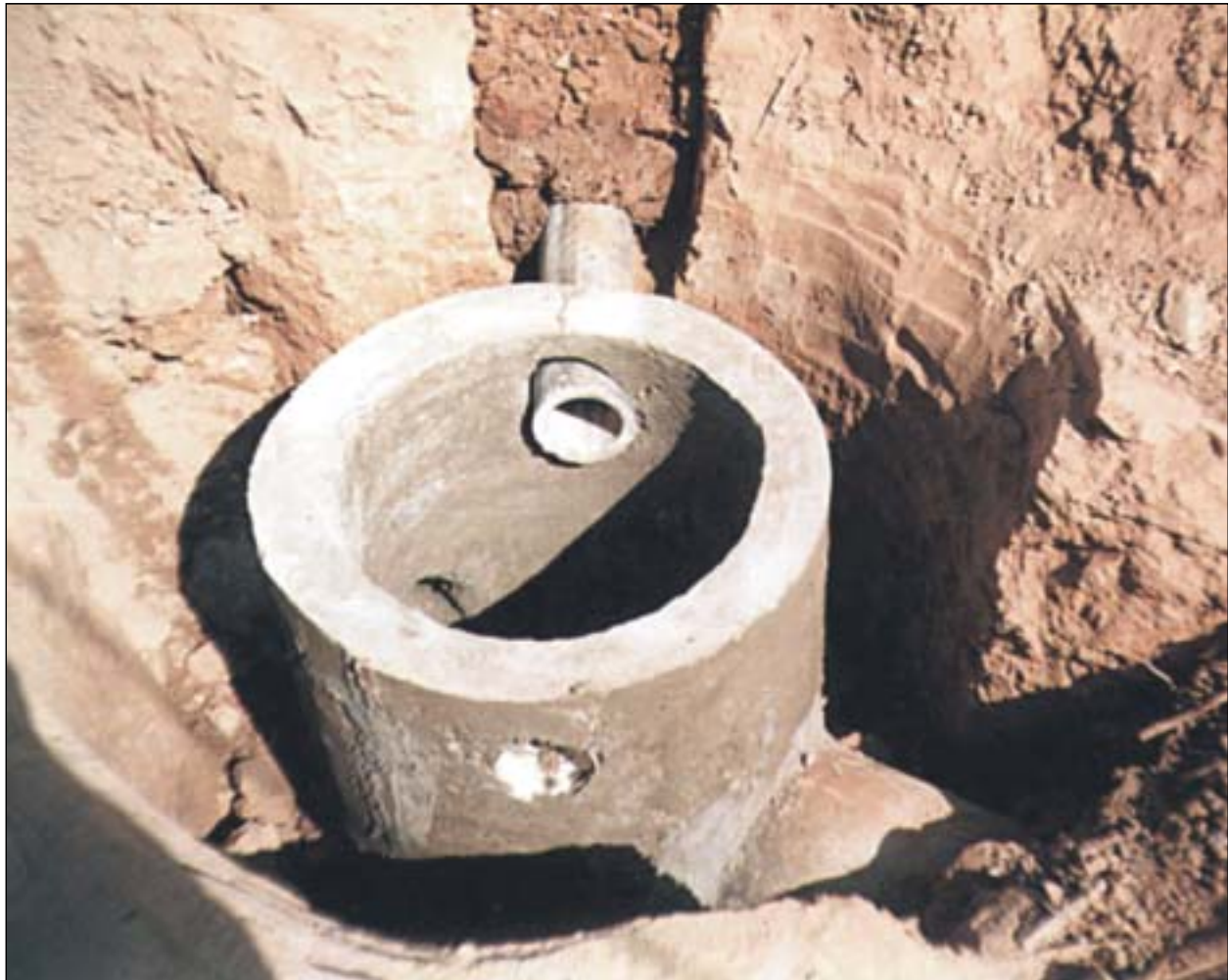
Figure 3-9 Concrete access chamber construction prior to backfilling
