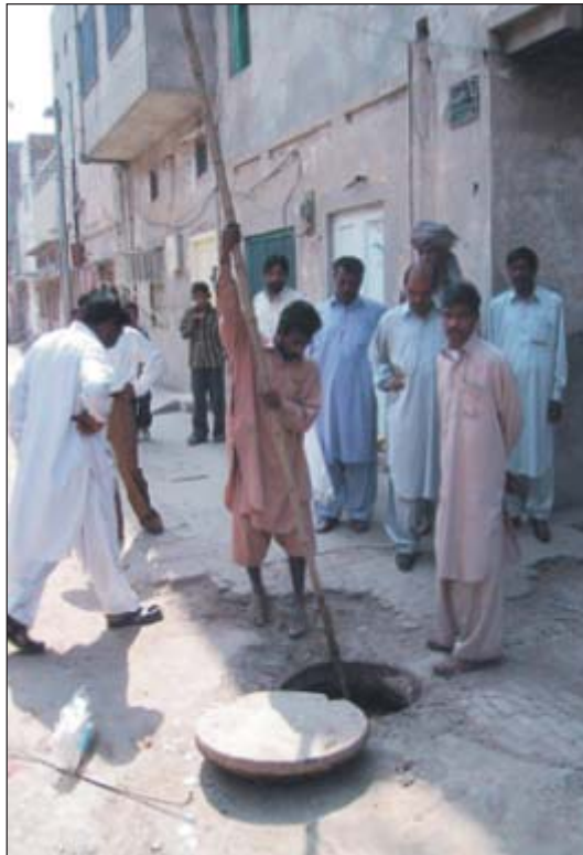
Figure 4-2 Cleaning sewers using wooden rods
