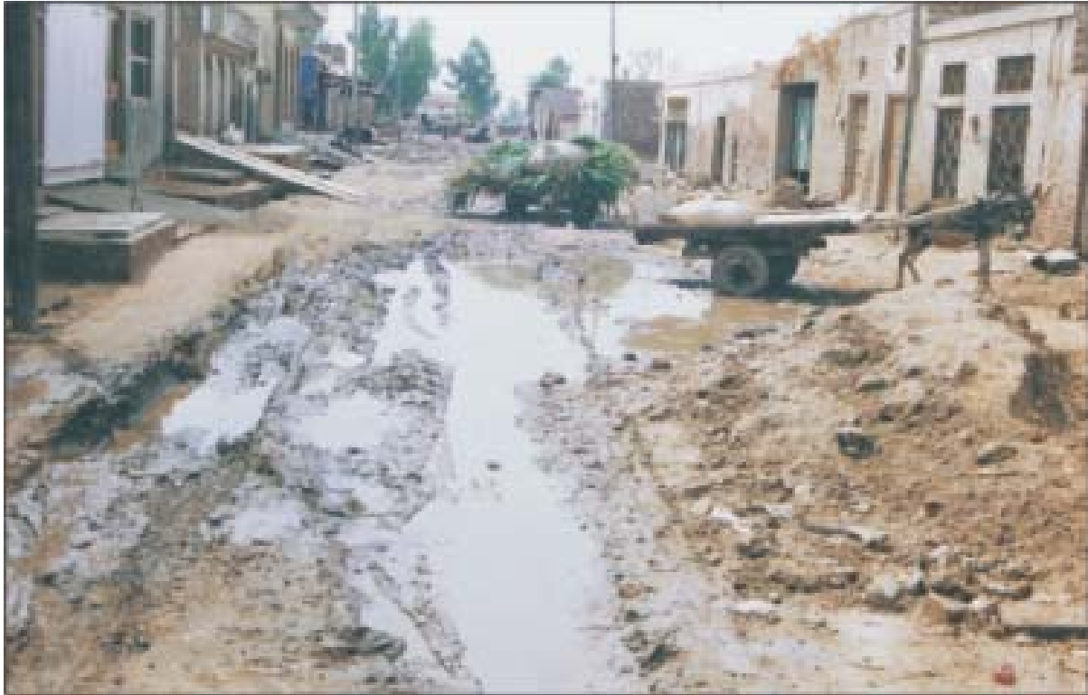
Photo: Condition prior to a secondary level sewerage project in NH-D
