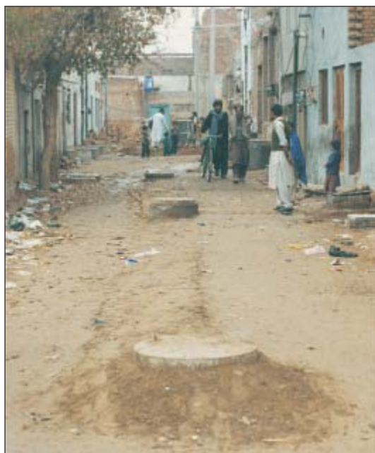
Photo: Communities insist on manhole spacing being limited to about 30 to 40 feet
