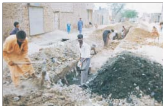
Photo: Community initiating a sewerage project
