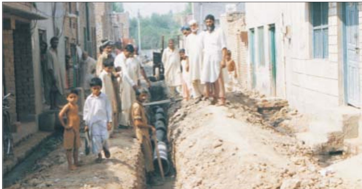
Photo: Community implementing a sewerage project
