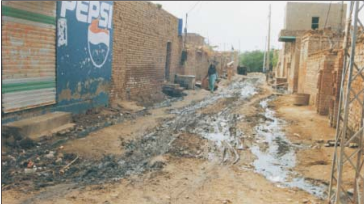
Photo: Before a community based sewerage project is implemented in Neighbourhood D
