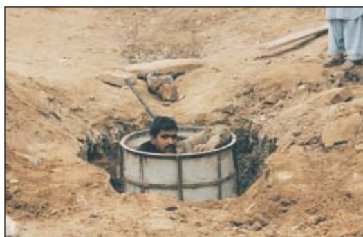
Photo: Construction of PCC circular manhole
