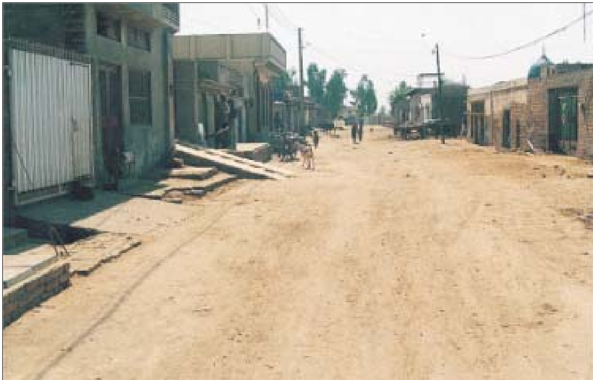
Photo: Condition after a secondary level sewerage project in NH-D
