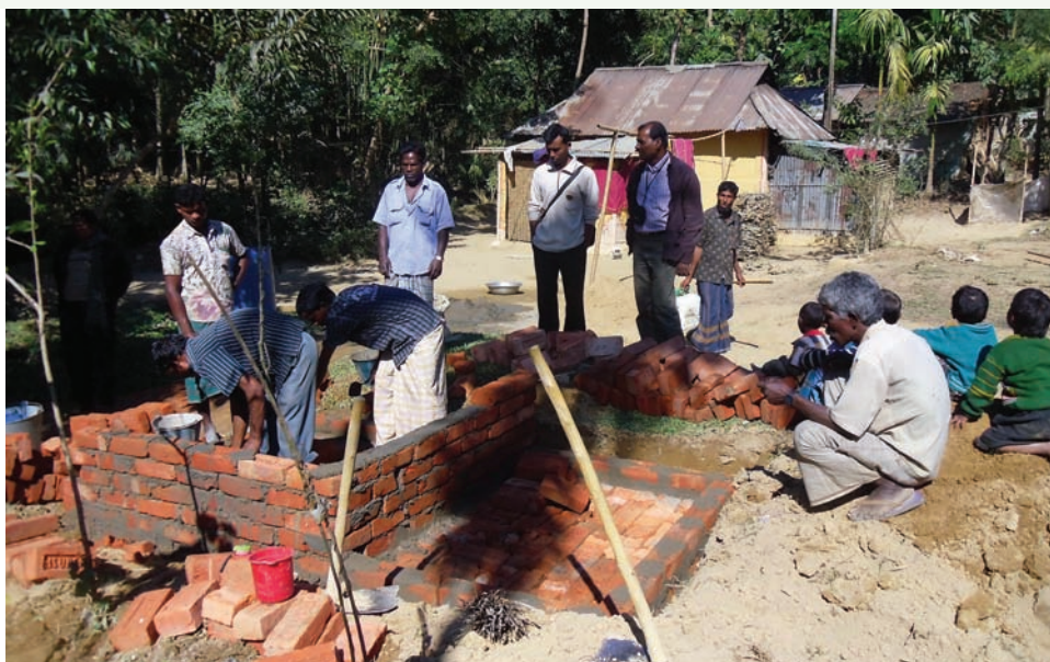
Figure 1 Hardware installation in the tea pickers' community WaterAid in Bangladesh
