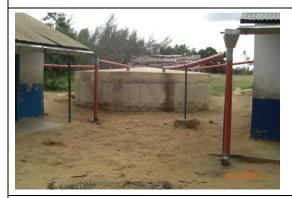
Concrete tanks use iron bars in foundation, walls and roof. The roof can be flat or inclined and needs a vent pipe. Wider tanks need a support pillar in the centre.
