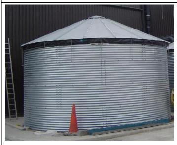
The outer part of these pre-fab tanks consist of iron sheets, that are put together with bolds and nuts. The inner side consists of a plastic lining with openings for the wash out and outlet pipes. Also the roof is from pre-fab sheets. The base needs to be stable.
