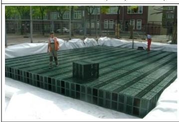
The modular crates, surrounded by strong foil, are meant to provide a solid subsurface below an area that can be used for a second purpose. The water tank can be used to store the water or to create a buffer for slower infiltration into the ground.
