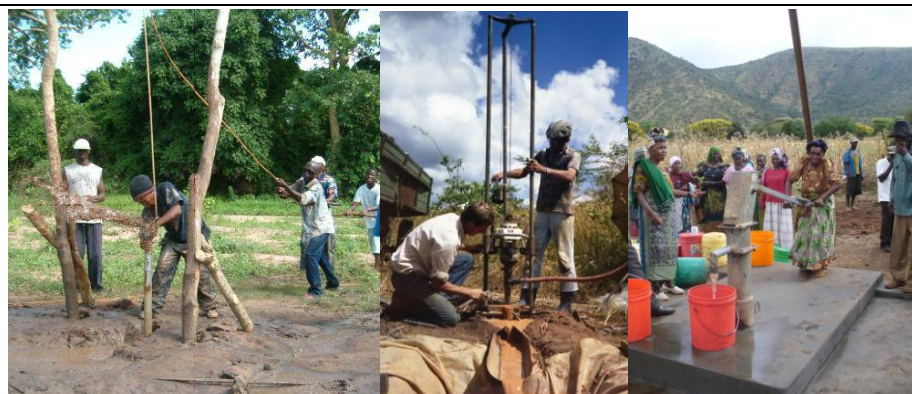
Baptist drilling (left) light machine drilling (middle) and pumping(right)
