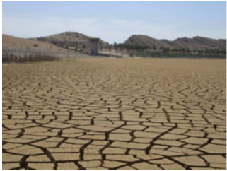
El-Houareb dam (Merguellil watershed, Tunisia) completely empty at the beginning of May, 2008 (photo Stephanie Guidon, IRD).
