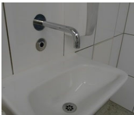
A tap with an infrared on-demand sensor.
