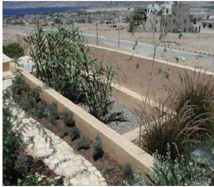
The wetland (filter bed) after 6 months of operation. The grass and bamboo started to grow.
