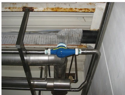
Installation of new water meters.
