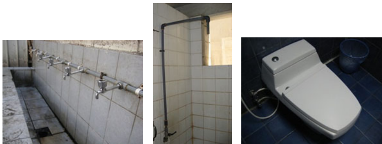
Typically encountered inefficient fixtures in buildings and facilities in the region.
