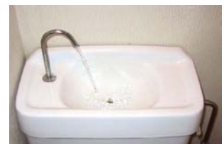
Water saving device on the Japanese toilet: Filling toilet flush tank while washing your hands. Source: Wikimedia Commons.
