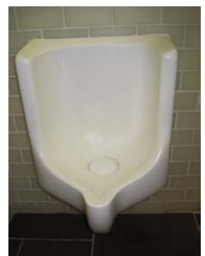
Example of a waterless urinal.
