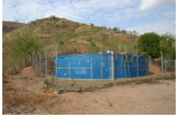
Storage Tank in Dili
