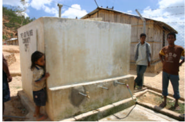
Community-Managed Scheme Missing Taps, Illegal Connection
