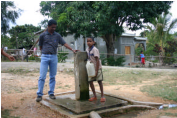
Community-Managed Scheme Functioning Tap Stand
