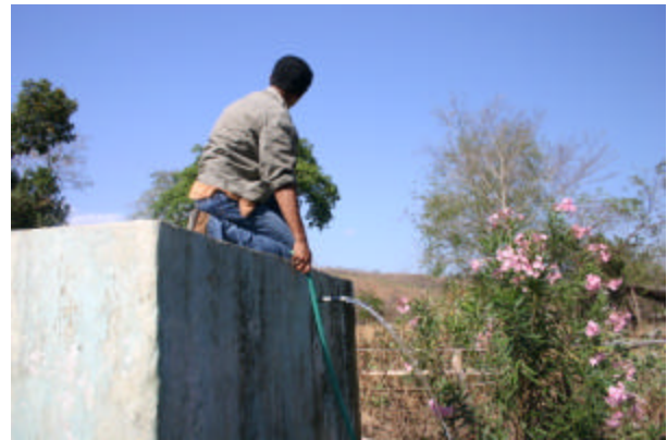
Community-Managed Scheme Illegal Connection from Overflow Pipe
