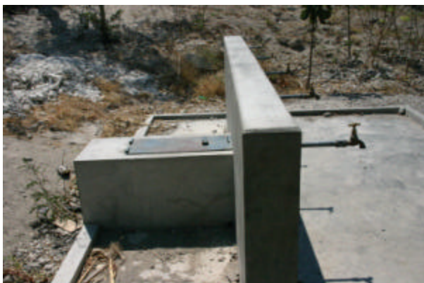
Tap Stand, Oecussi Showing Box with Meter, No Water
