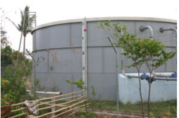
Empty Storage Tank, Maliana
