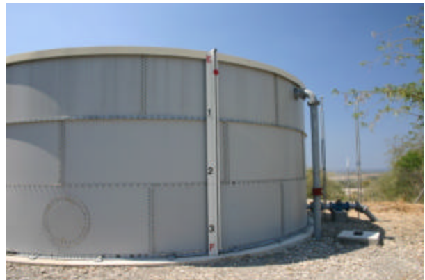
Empty Storage Tank, Oecussi
