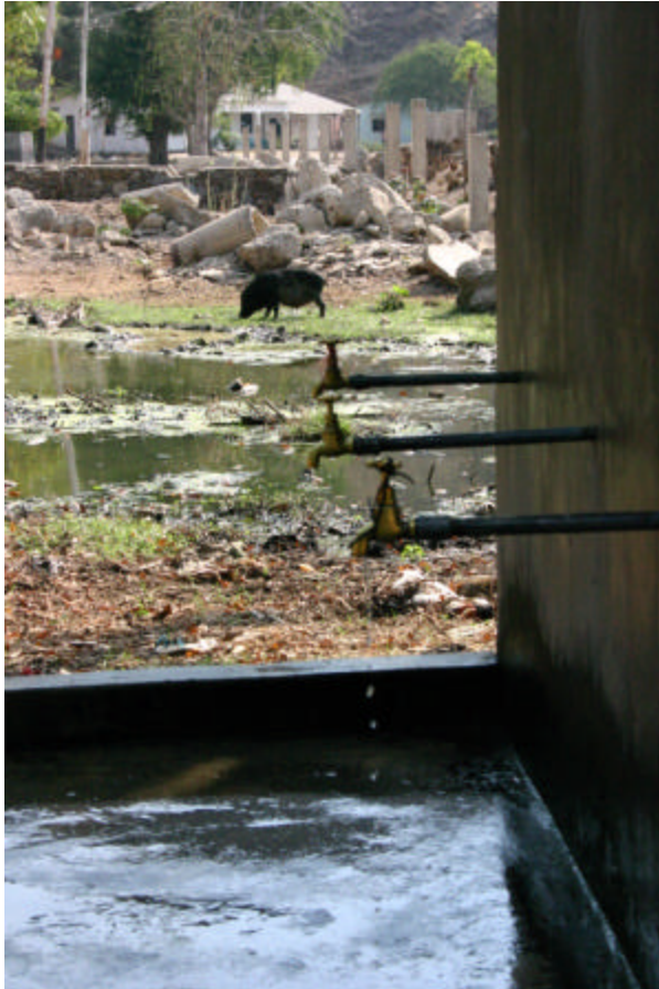
Public Tap Stand in Dili Area Showing Leaking Taps, Poor Drainage, and Animal Presence
