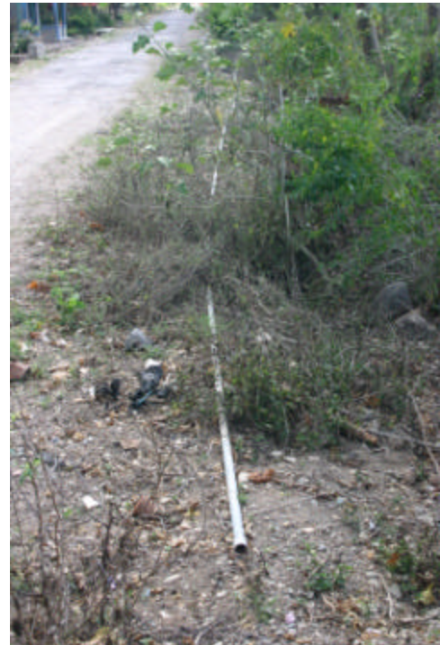
Community-Managed Scheme Pipes Removed
