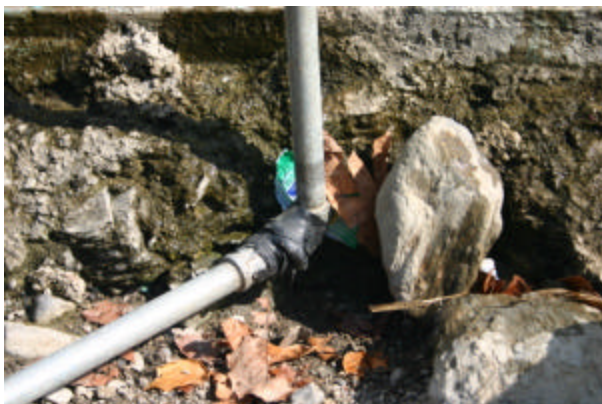
Community-Managed Scheme Control Valve Removed
