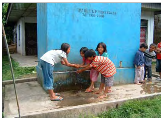
Working public hydrant
