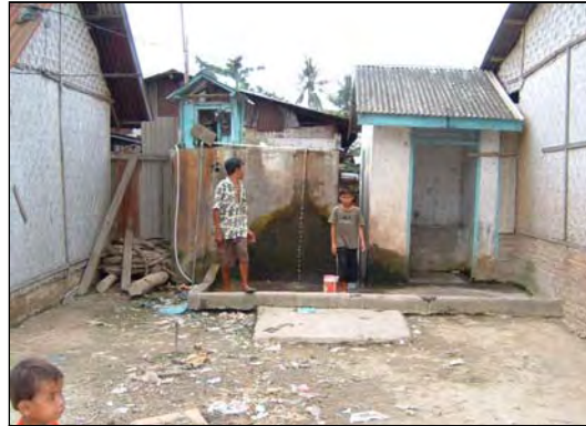
MCK within 1 meter of a shallow well
