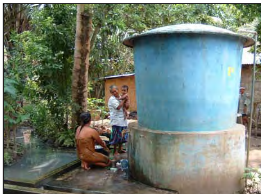
Public hydrant—note the poor drainage
