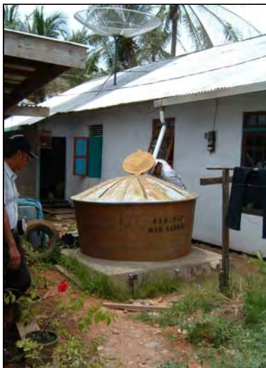
Rainwater harvesting tank
