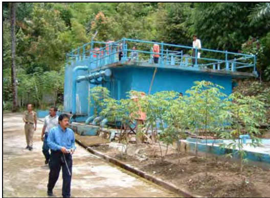
Treatment plant—note site well maintained
