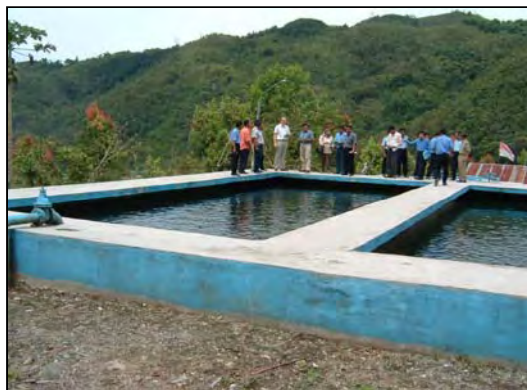
Slow sand filters—note good construction
