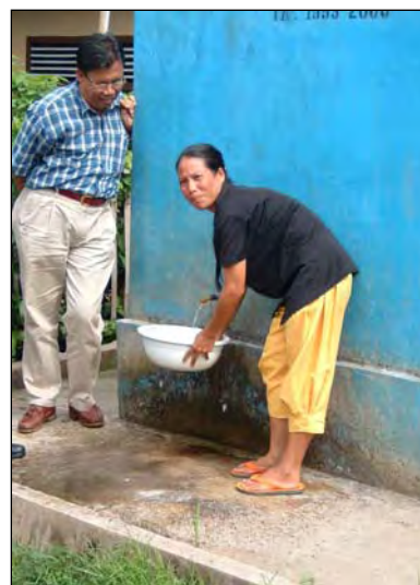
Working public hydrant
