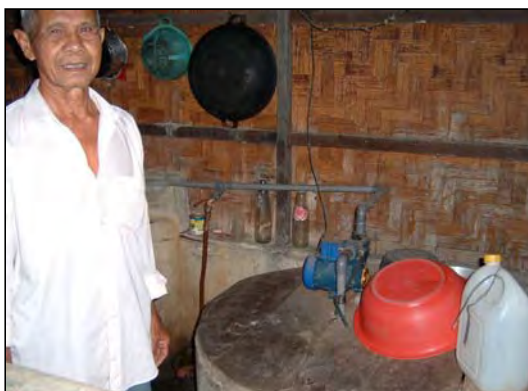
Private shallow well and electric pump
