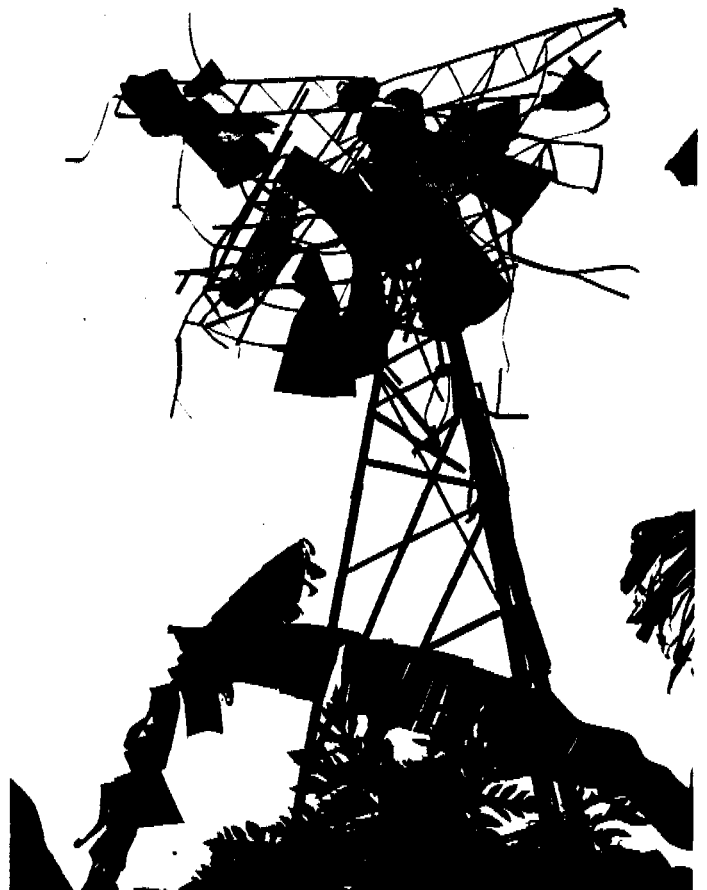
Fig 15 Windmill damaged by hurricane Isaac, 1982.
