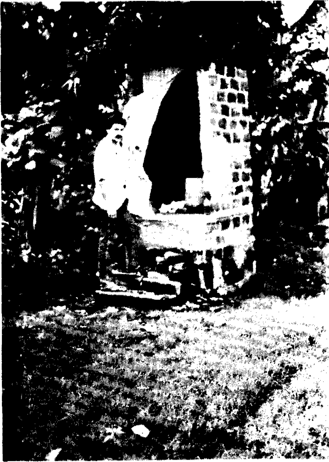
Photo 1: Household elevated unvented latrine in high groundwater area. Not effective in avoiding groundwater contamination.
