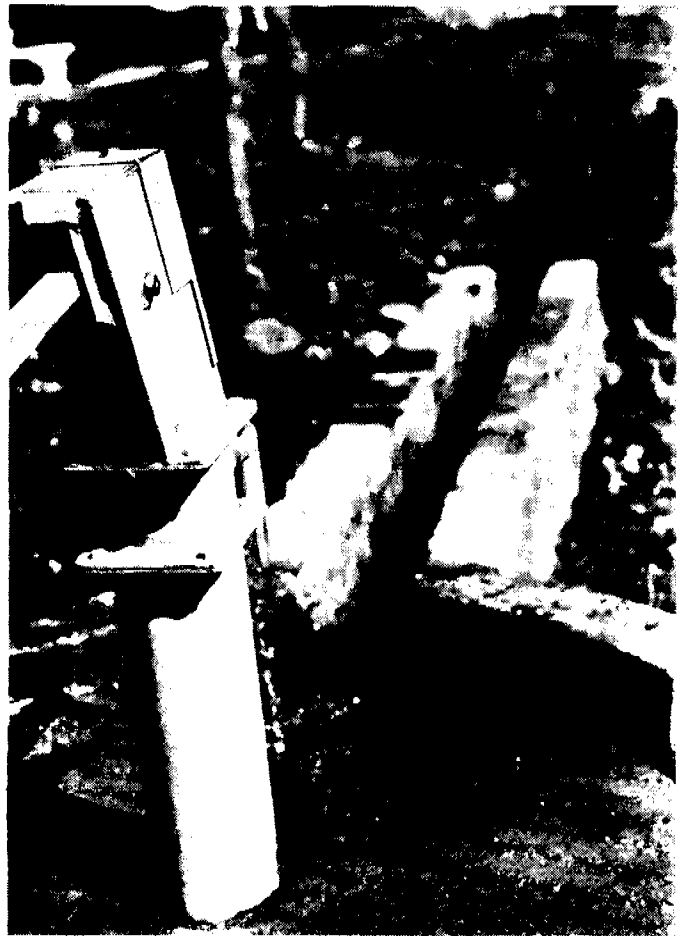
Photo 6. Handpump at the community house. Note poor drainage system and water pools.
