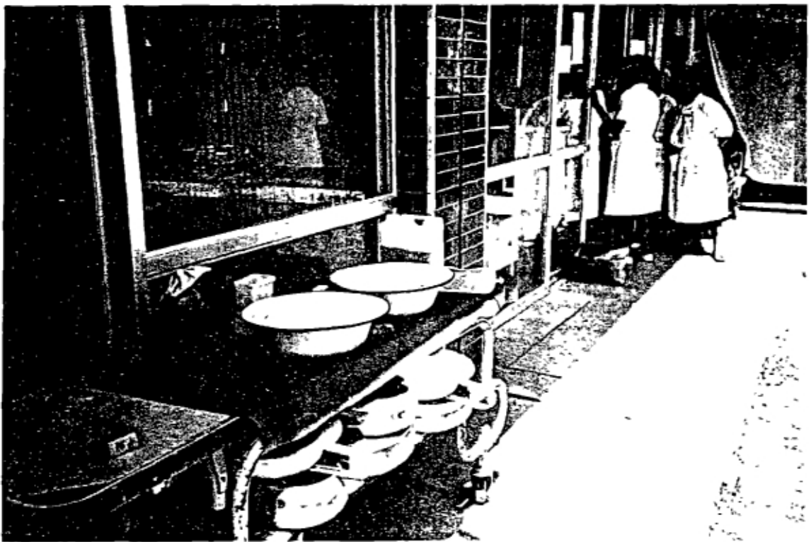
Bed Pan Disinfection Station Regional Hospital—Piura
