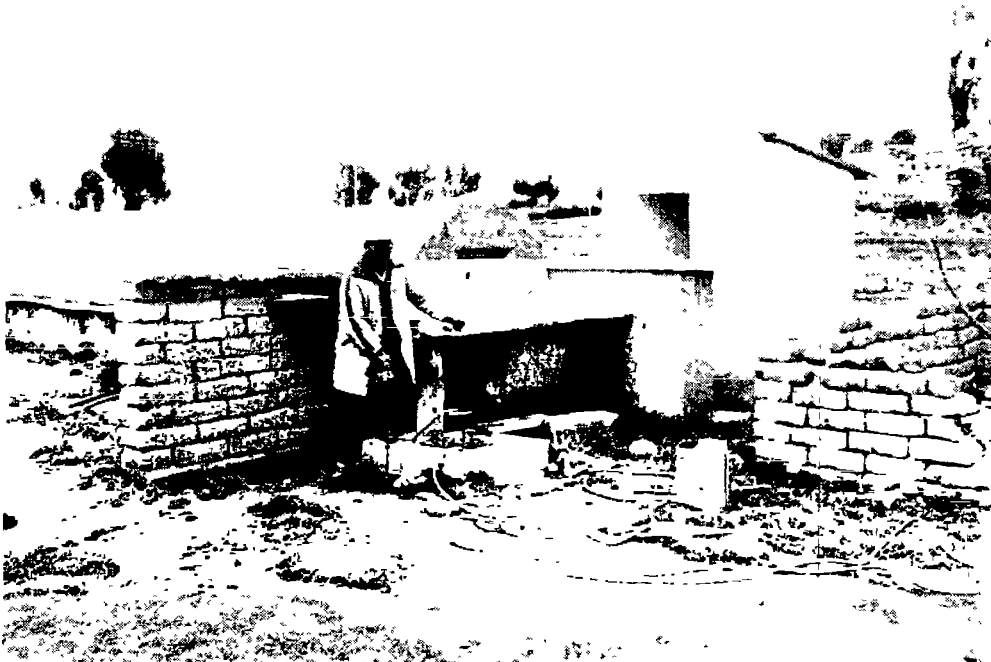
Photo 11: This combination of a yard tap, wash basin, and latrine in the village of Compi, La Paz, is one of the most popular options the project offers to beneficiaries. The hose in the foreground and the greenhouse in the background point to the very common use of domestic water for garden irrigation, even though the systems were not designed to supply enough water for this purpose.
