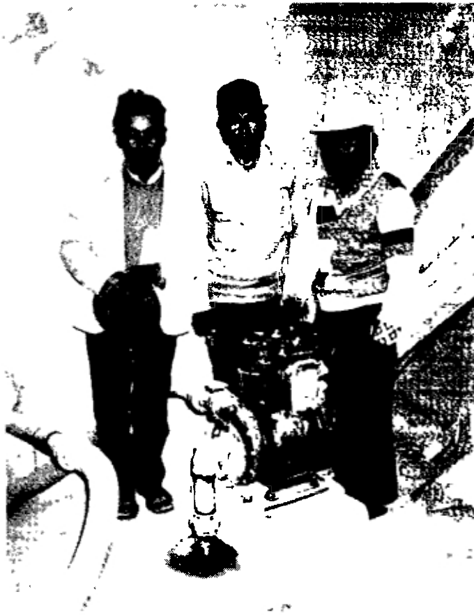
Photo 20: This photo shows the motorized pump in the village of Nueva Llaguas, Oruro. Although this pumped system has no technical problems, the villagers can only afford to pay a monthly tariff of one Boliviano ($0.33), and as a result there is only enough diesel fuel to provide water for about 45 minutes a day. The operation and maintenance cost of motorized pumps is a problem for the few such systems the project has constructed.
