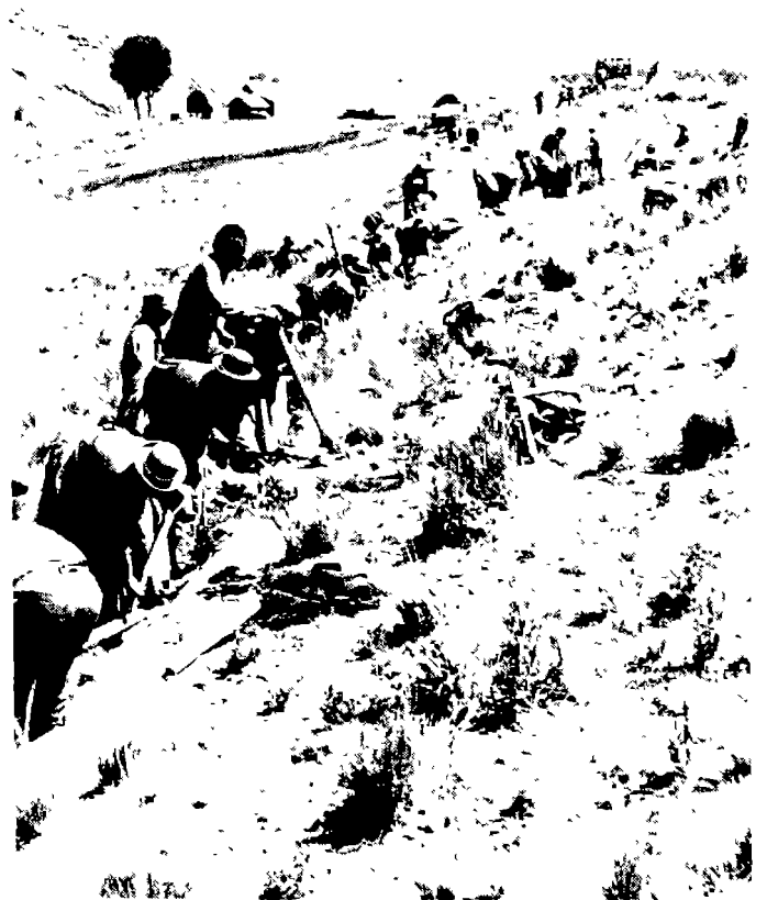
Photo 6: The whole community, women as well as men, has turned out in Ajlla Pata Pata, La Paz, to work on construction of their long-awaited water system. Construction was delayed nearly three years while this community worked out an agreement to share a water source with another community
