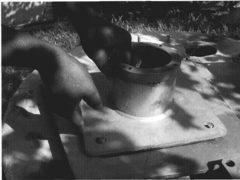
2. Place the base plate on the gasket.
