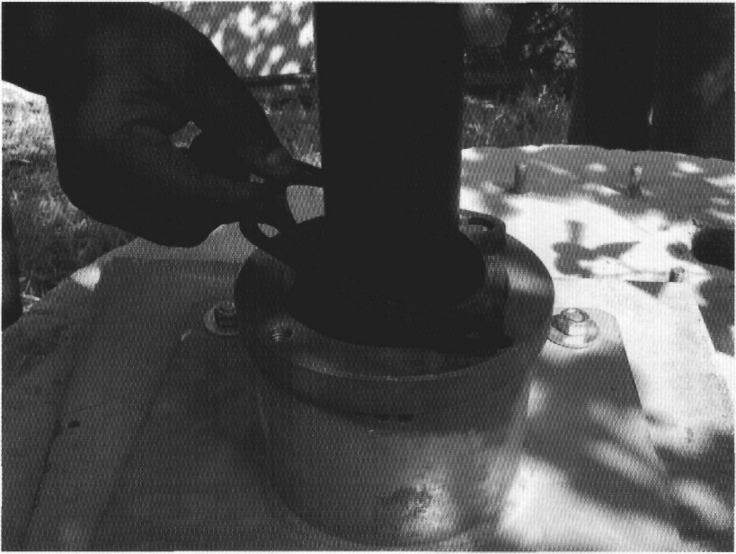
7. Place the smaller gasket on the base plate.
