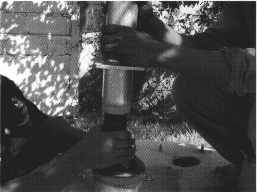
8. Connect the pump stand on to the last riser pipe.
