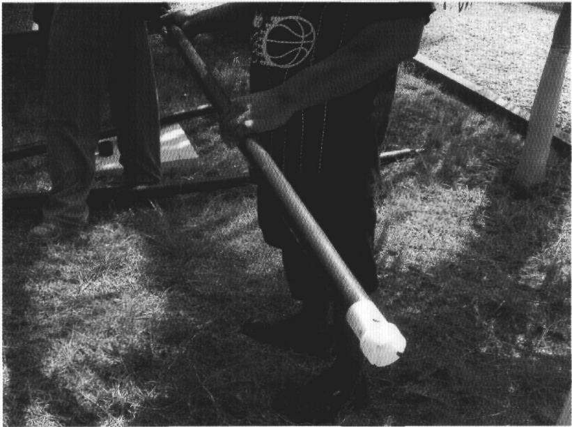
12. Connect the plunger rod to the pump rod.
