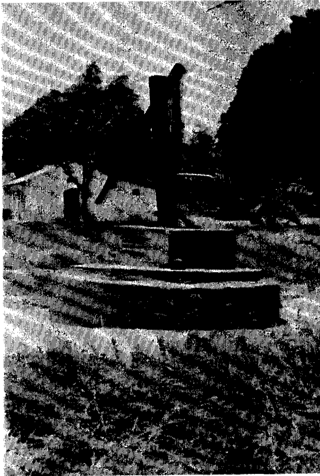
Fig. 3.22 Shinyanga pump on old shallow well (Tabora Region)
