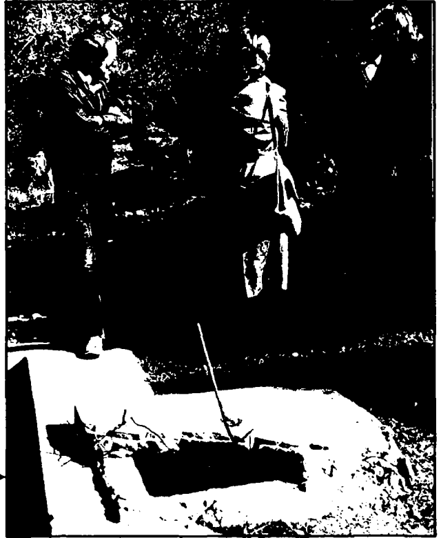
Springs were improved at 139 sites so that the water would flow through a pipe and into a concrete trough.
