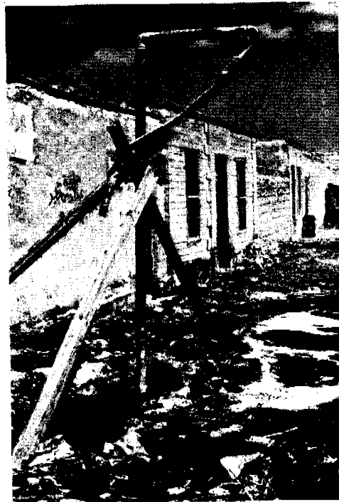
Unsanitary conditions at tank truck filling station.
