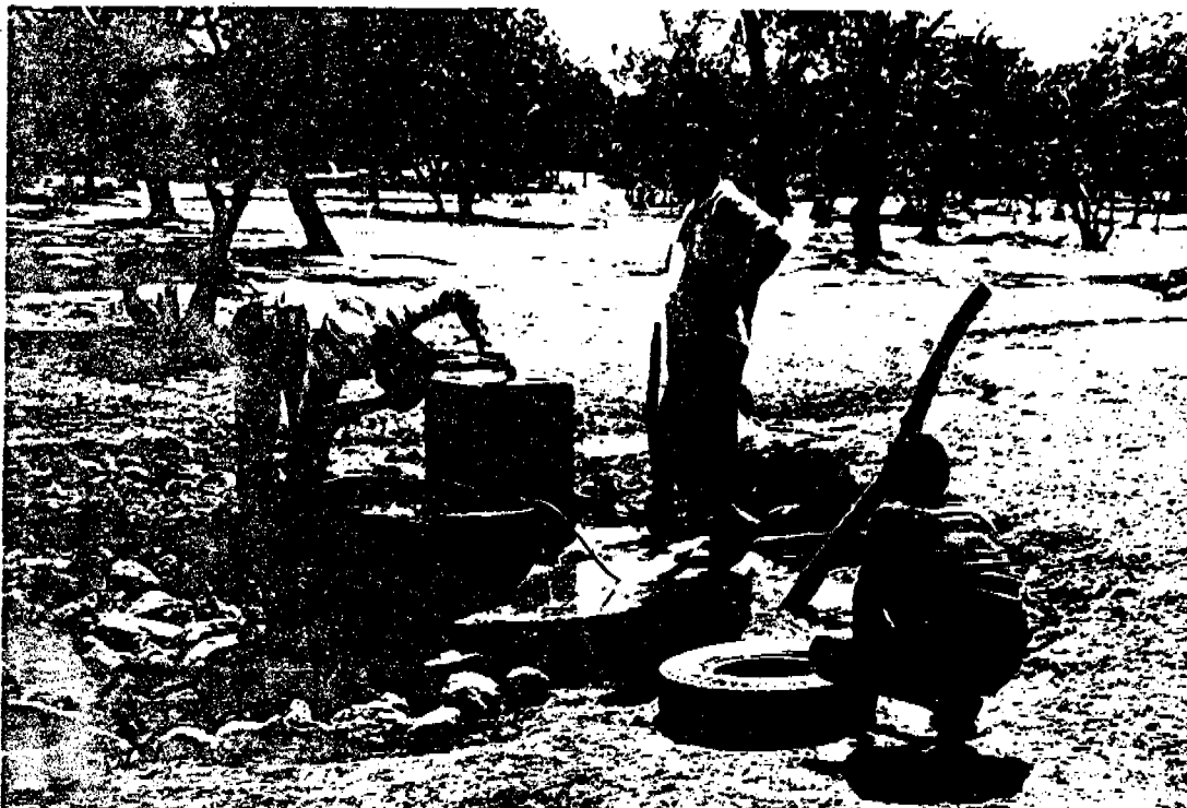
Maganyani Piped Water Supply: mending a tyre at one of the standposts. The soil erosion and lack of a fence are signs of poor village-level maintenance .
