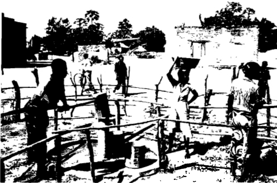
Photo 4: India Mark II handpump with fence
